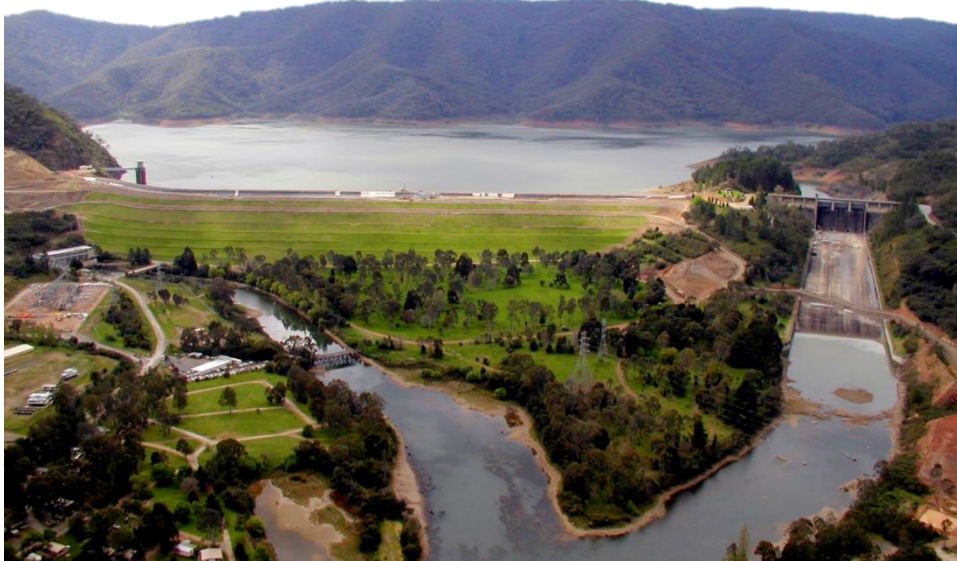
Eildon Dam in Victoria, Australia. Taken during dam safety upgrading works
