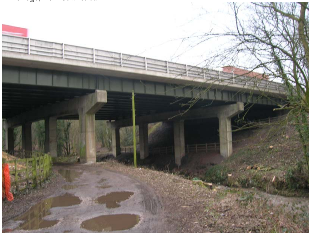
AX bridge, from downstream
