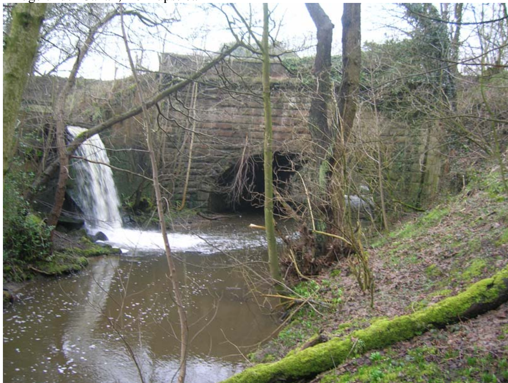
Bridge under Canal , from upstream
