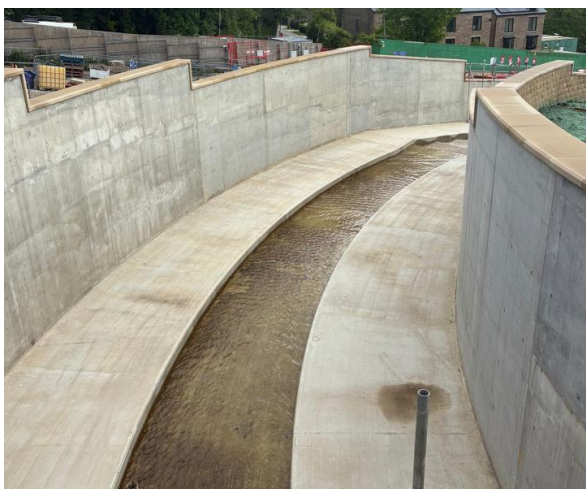
Figure 2 New Auxiliary Spillway under low flow conditions
