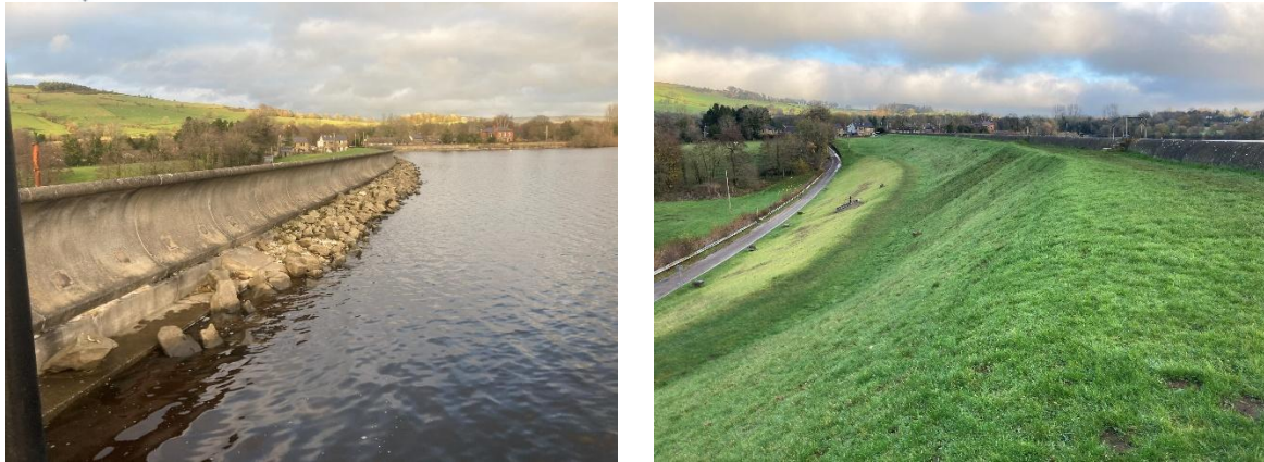
Figure 4 Combs Reservoir – Concave wave wall and stability berm
