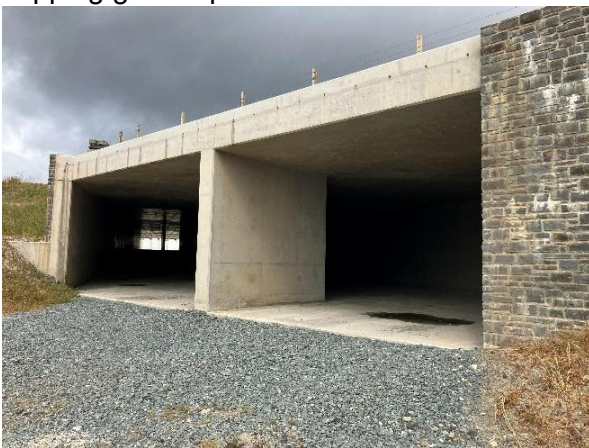
Culvert discharge point
