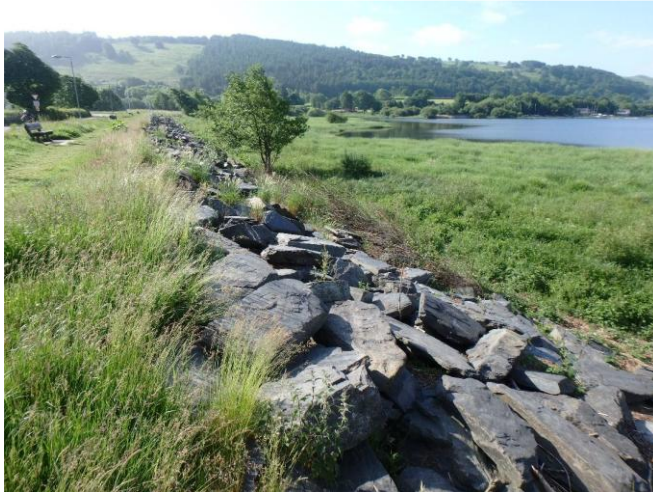
Figure 7 - Lake Embankment original slate Rip Rap
