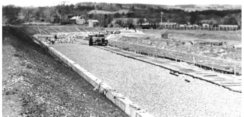
Approach channel to Weir X
