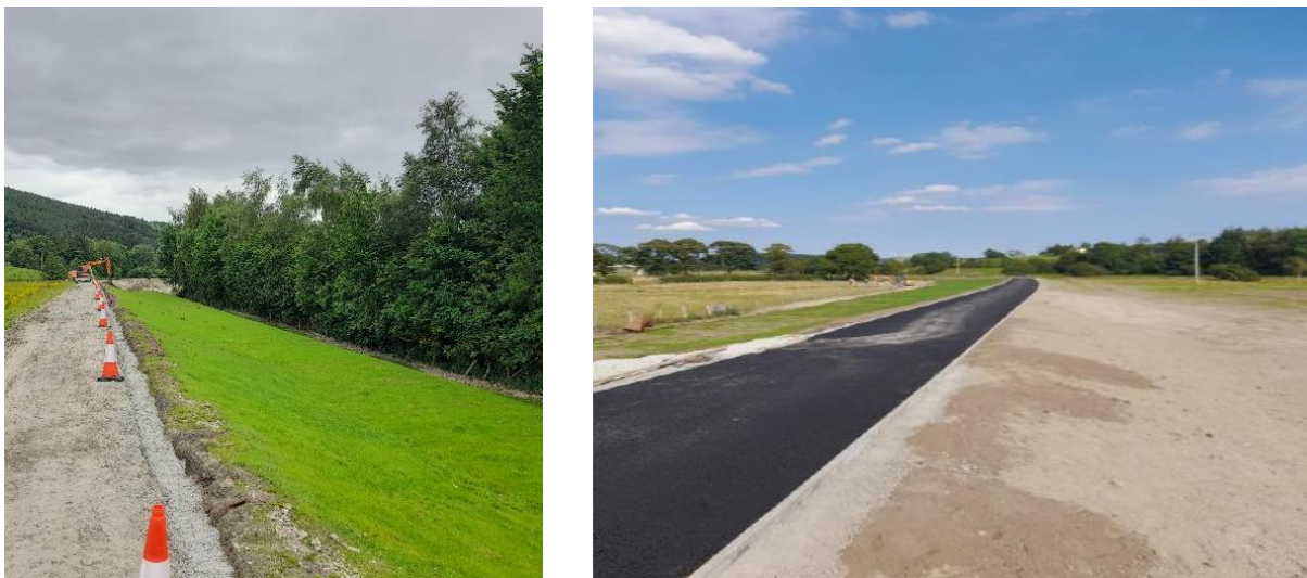
Figure 11 - TRM grass uptake and footpath installation
