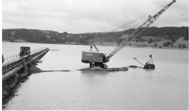
Lowering the lake level by 7ft
