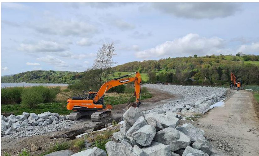
Figure 8 - Lake Embankment Rip Rap works 2022
