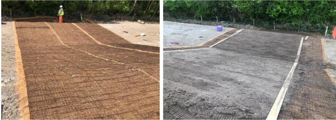
Figure 10 - River Embankment showing TRM installation
