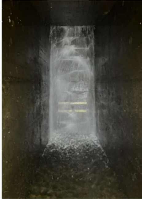
Figure 13: Downstream Face of the Upstream limpet Cofferdam
