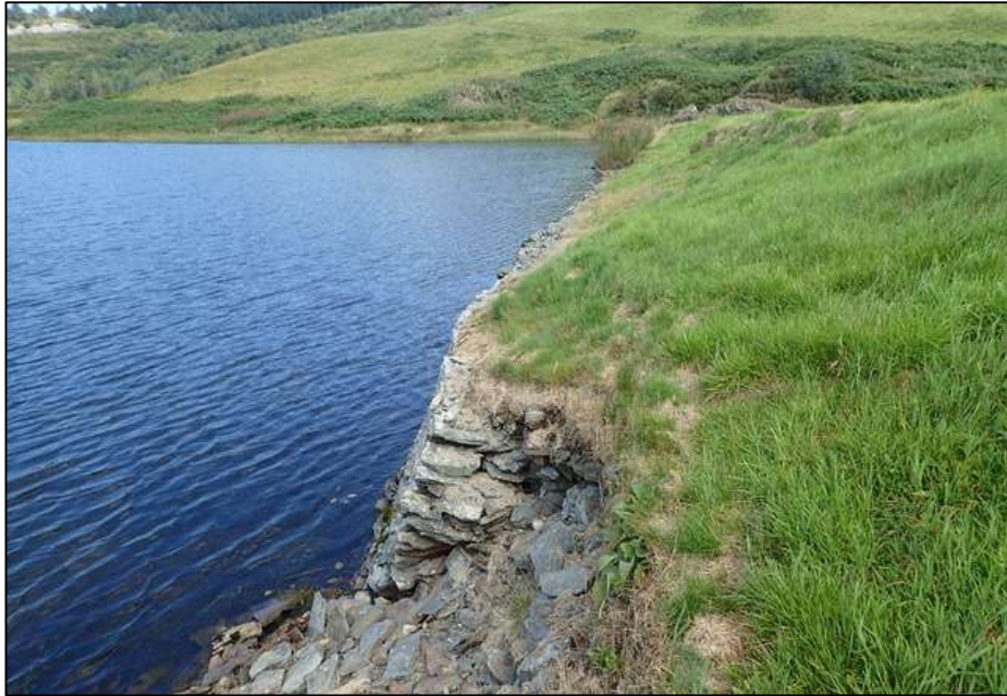
Figure 3. View along the dam at Llywernog Pond
