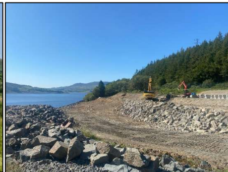
Figure 19. Enabling works at the new spillway location
