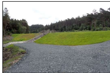
Figure 5. Pandora Reservoir in 2024 following completed capital works
