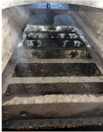
Figure 15: Scour Gate in Position Prior to Removal
