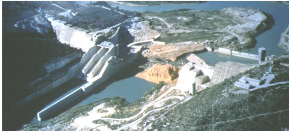
Figure 3. Tous Dam after failure in 1982. Source: Fleitz, J. (2013).
