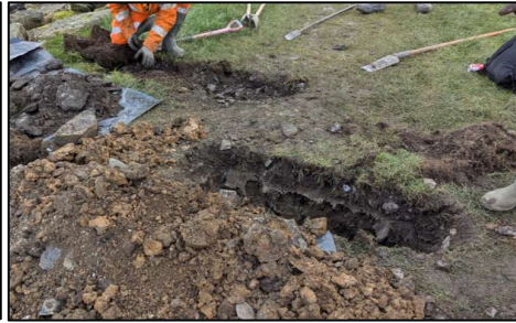
Figure 22: Excavation of a slit trench at Lower Foulridge.
