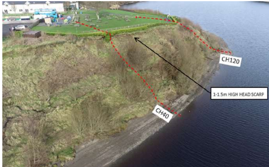
Figure 6. View of slopes before works
