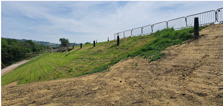
Figure 5c Several temperature soundings, covered by telemetry pillars, along the downstream side of the dam crest
