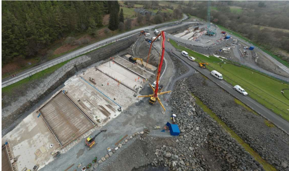
Figure 21. Reinforced concrete bases under construction upstream and downstream of the dam core
