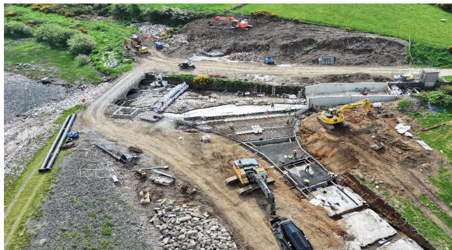
Figure 9. Phased Spillway Construction
