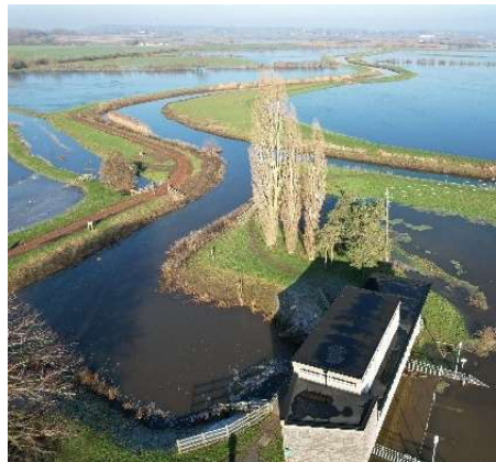
Figure 2. Westmoor Reservoir under flood conditions.
