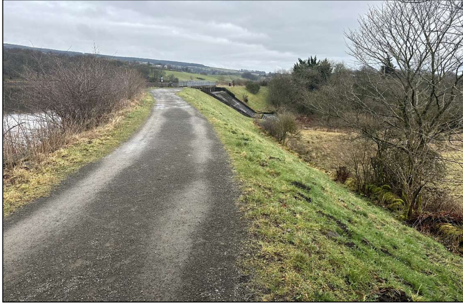
Figure 5. Crest and Downstream Face of Embankment
