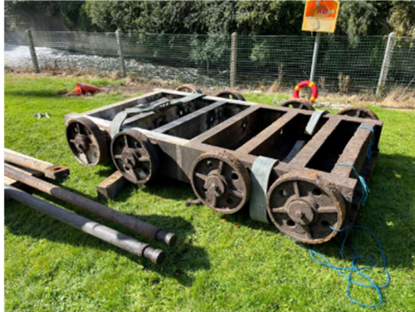
Figure 16: Scour Gate Removed and Ready for Transportation
