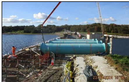
Figure 2. Installation of pipes through dam, to priming chamber (Oct 2024)
