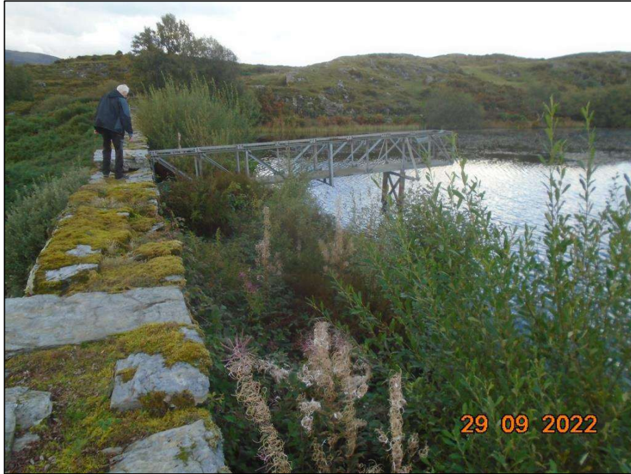
Figure 2. The elderly Undertaker inspecting Llyn Ffrith Carreg y Bwch Reservoir dam, precariously perched on the narrow crest
