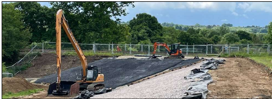
Figure 4. Installing OSA between the control structure and the railway in the north spillway section.
