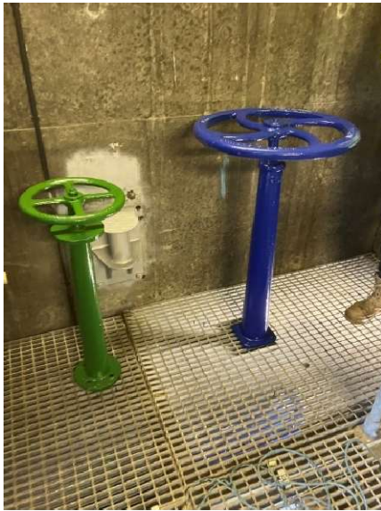
Figure 2. Painted Valve work in Valve Chamber
