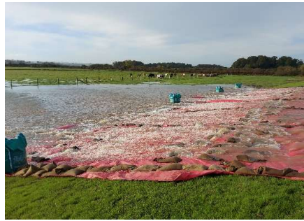
Figure 5. Temporary winter slope protection measures in operation.
