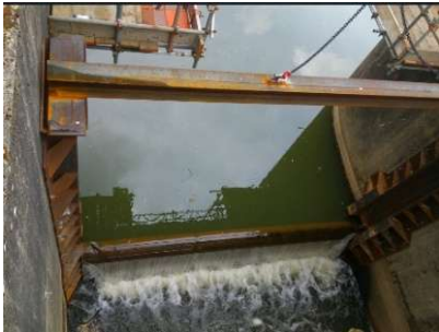
Figure 7. Low flow stoplog weir.
