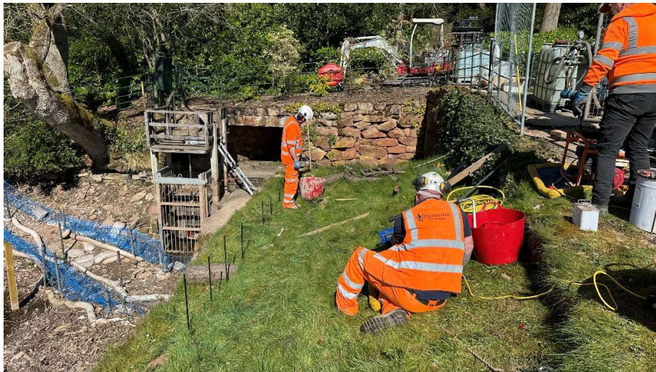
Figure 5. Polyurethane resin injection at the upstream crest to reduce permeability across the presumed infiltration zone for seepage.
