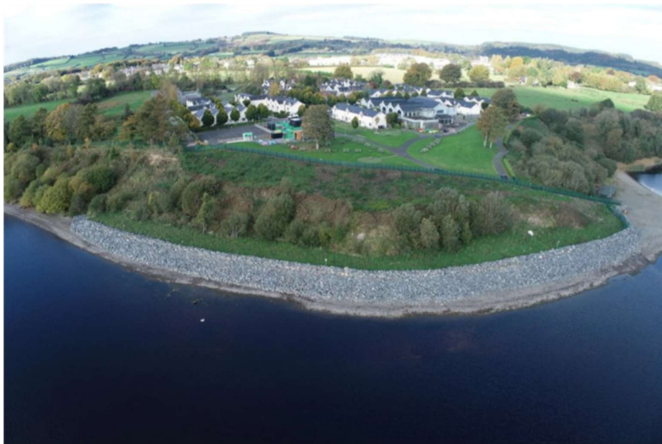
Figure 13. Aerial view of completed works
