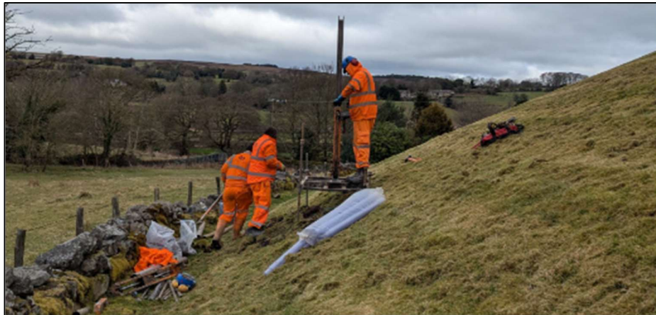
Figure 4 - Mott MacDonald GI at Lower Foulridge Reservoir
