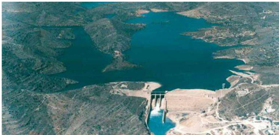
Figure 1. Tous Dam before the failure. Source: ICOLD (n.d.).
