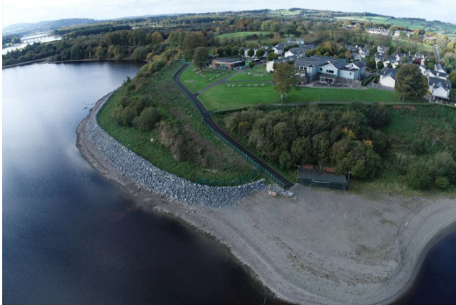
Figure 12. Aerial view of completed works
