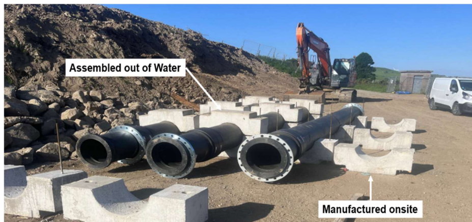
Figure 10. Siphon Pipe Preparation
