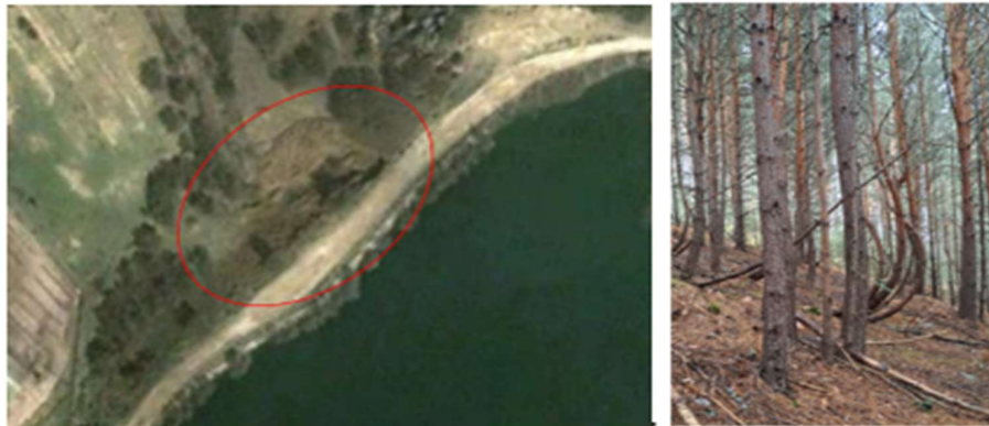
Figure 2. Slope instability and dense vegetation on the downstream slope
