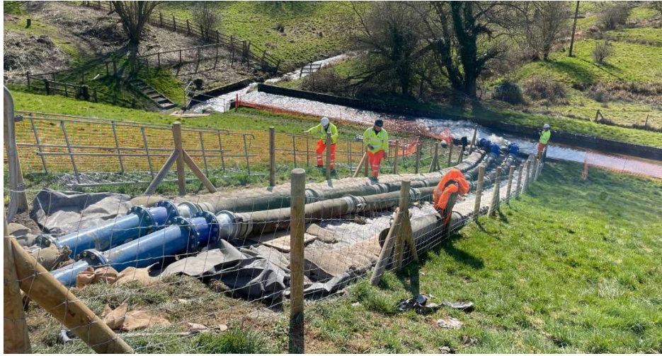
Figure 7. The finished syphon (looking downstream)
