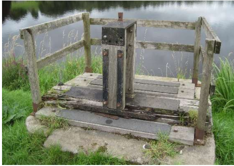
Figure 4 – Slipper Hill upstream masonry wetwell at low level outlet
