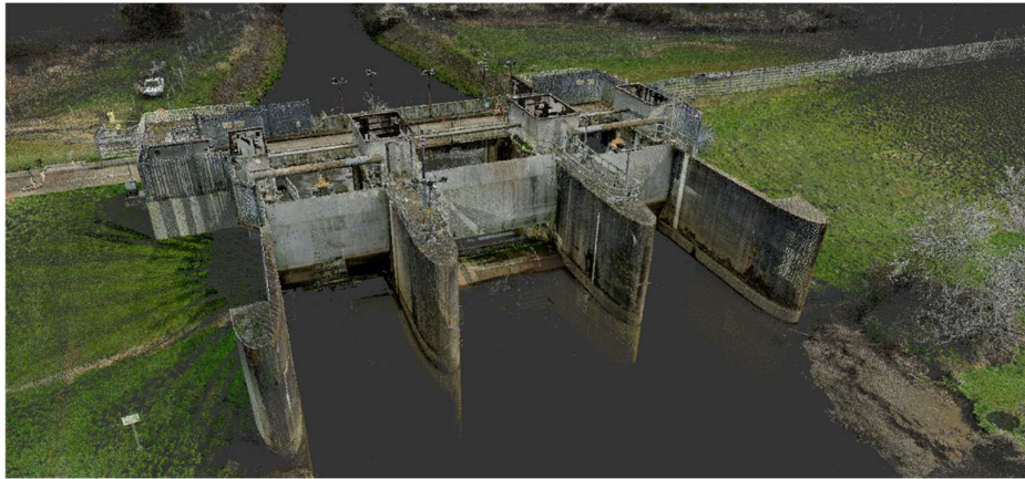
Figure 9. 3D laser scan & photogrammetry survey.
