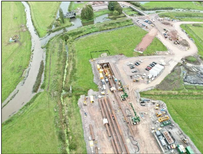
Figure 11. Temporary works – Pile layout area and plant
