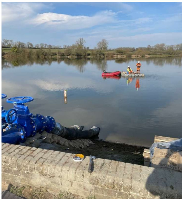
Figure 8. The finished syphon (looking upstream)
