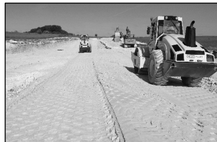
Figure 4. Compaction using both padfoot and smooth rollers
