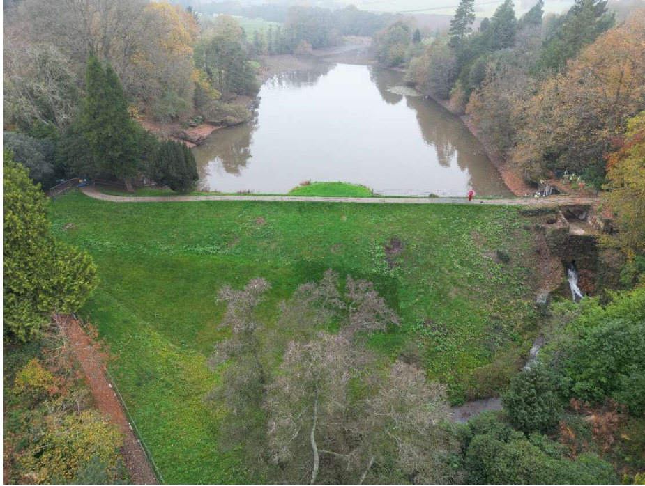
Figure 1. Overview of the dam embankment and reservoir. The overflow and outlet works are located at the left abutment (right side as viewed).
