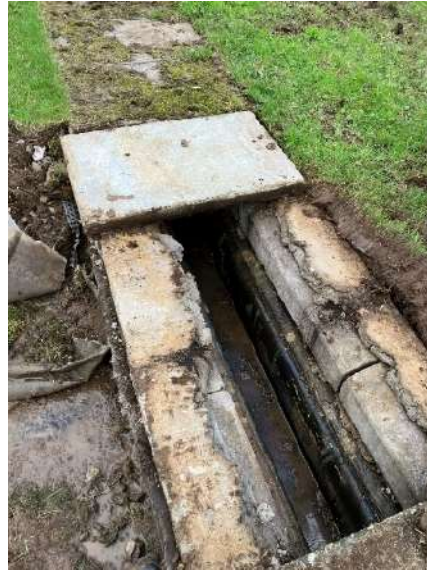
Figure 11. Exposed Central Roof Trough
