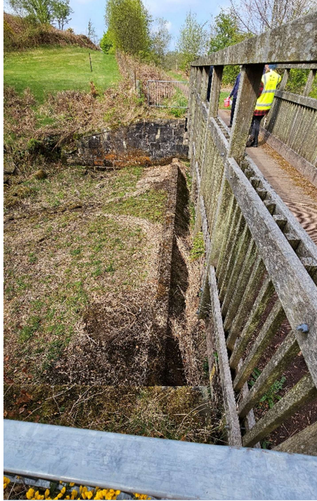
Figure 2. Main Concrete Weir
