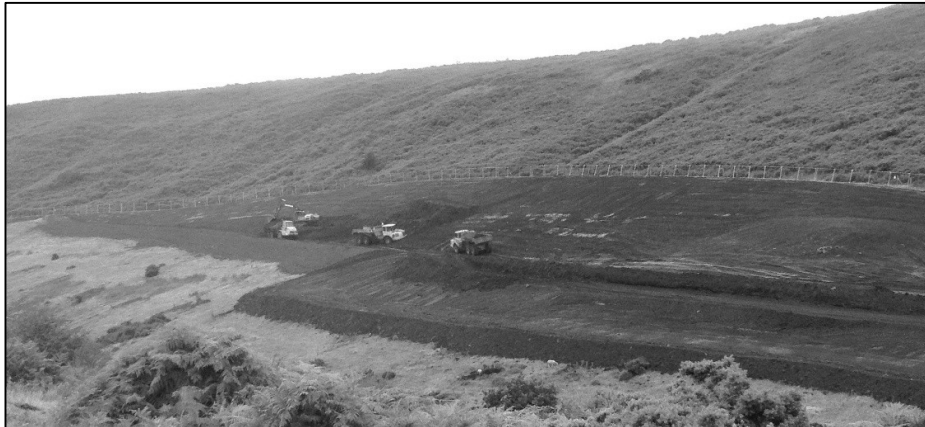
Figure 9. Colliery spoil being sourced as fill for the embankment dam
