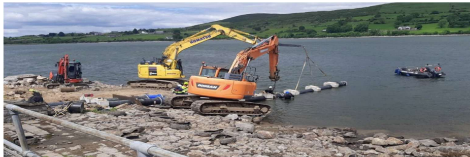
Figure 11. Siphon Pipe Installation
