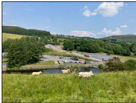
Figure 18. Enabling works from the hydraulic right side of the valley
