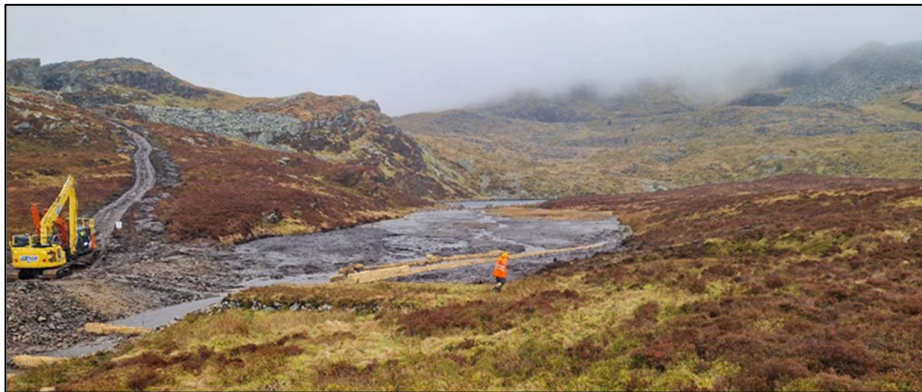
Figure 7. Completed drawdown and dam removal with silt mitigation and silt retention measures being added
