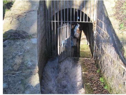
Figure 5 – Slipper Hill downstream masonry portal at low level outlet
