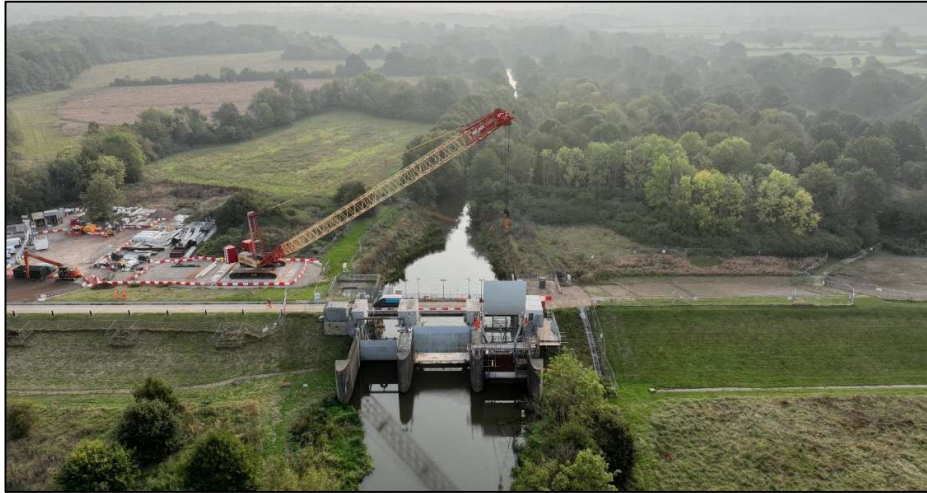
Figure 11. South gate leaf installed by a 300t crane.
