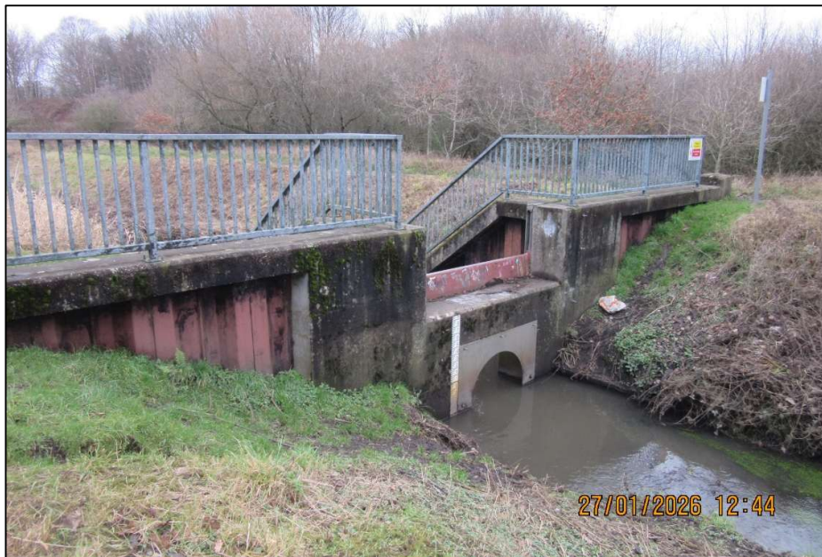
Figure 4. Timperley Brook FSB – In-Channel Control Structure (MM, 2026)
