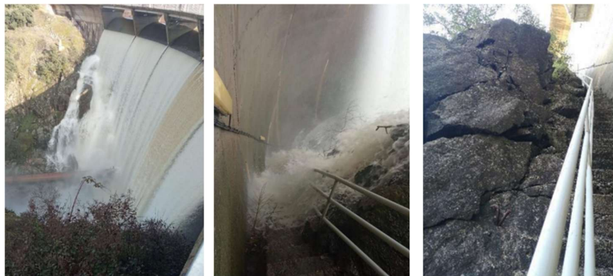
Figure 8. V Spillway discharge over abutments and access staircase to the bottom outlet
