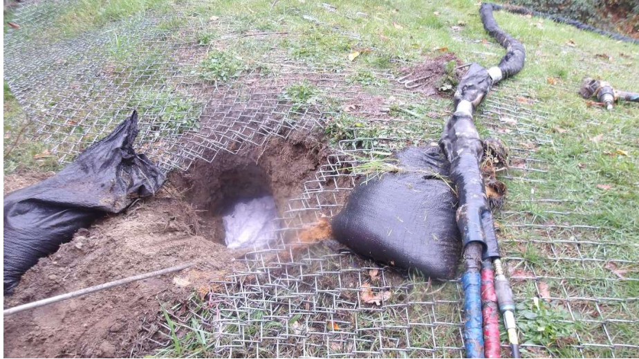
Figure 7: Resin expanding to fill sett
