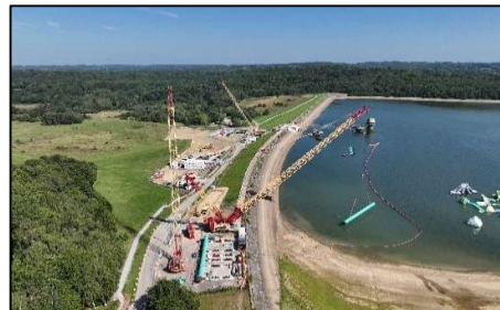
Figure 3. Lifting and floating of marine side pipes (Aug 2025)
