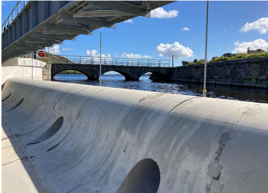
Figure 7. Spillweir Penstocks
