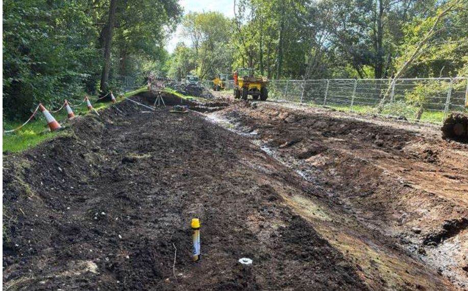
Figure 4. View of section of old bund (left) and new embankment construction with additional key trench into foundation (right)
