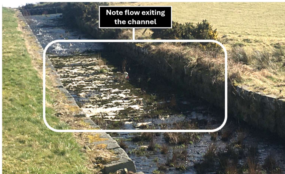
Figure 3. Spillway Deterioration
