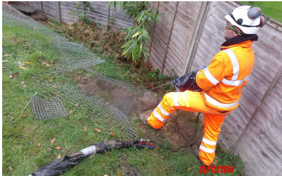
Figure 6: Pressure injection of resin into centre of sett
