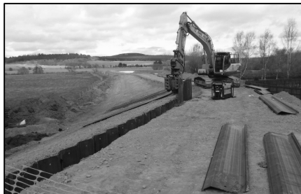
Figure 6. Installation of sheet piles
