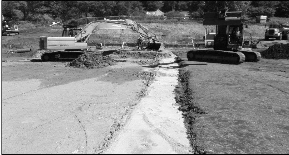
Figure 10. Chimney drain between core (left) and downstream shoulder
