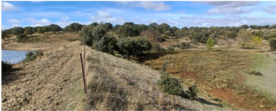
Figure 6. Seepage through the foundation
