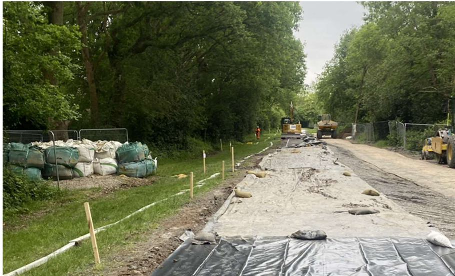
Figure 5. View of section of work with bulk bags ready for installation
