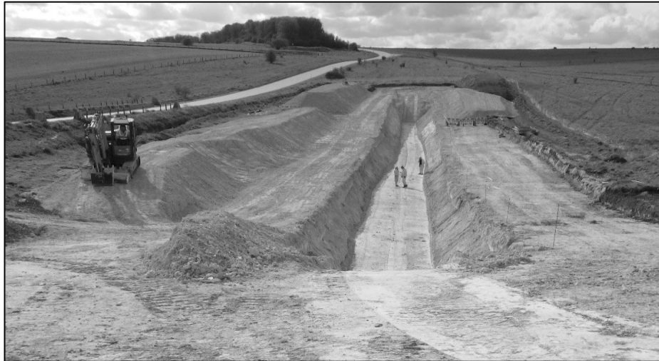
Figure 2. Inspection of cutoff trench, note the prepared stockpiles of excavated chalk intended for re-use
