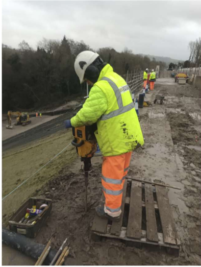
Figure 5a Ramming of a temperature sounding steel tube at Toddbrook Reservoir
