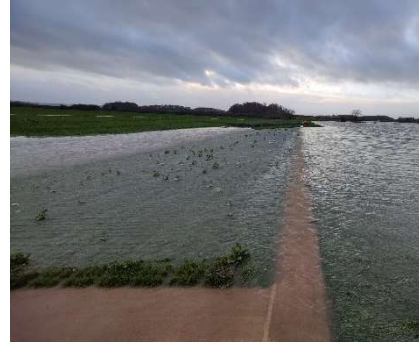
Figure 7. Isle Spillway in operation in winter 2025.
