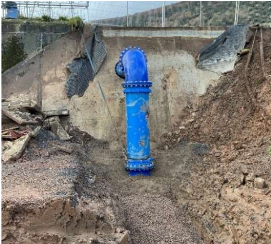
Figure 8. External Overflow Installation
