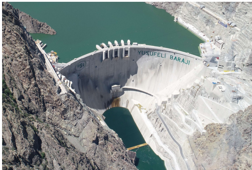
Figure 12: Yusufeli Dam on first impoundment
