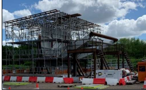
Figure 8. Gate assembly jig and scaffold for enclosure on site.
