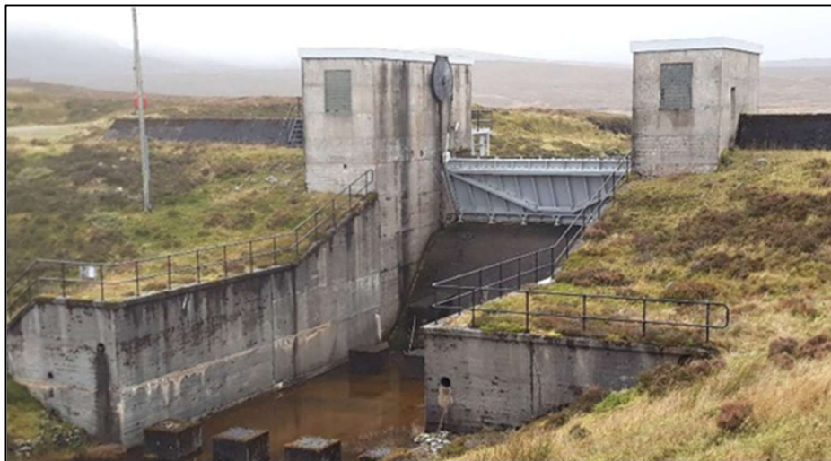
Figure 1. View of Liath dam and gate from downstream
