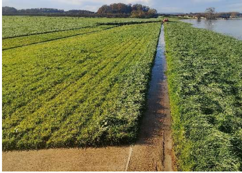
Figure 6. Isle Spillway reinforced with Dycel blocks in December 2025.
