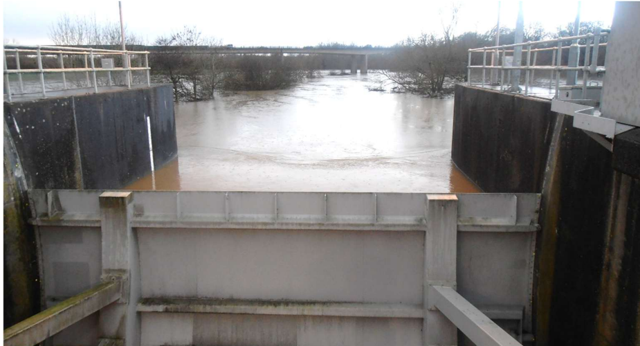
Figure 2. Peak water impounded upstream of the control structure during the December 2013 floods.
