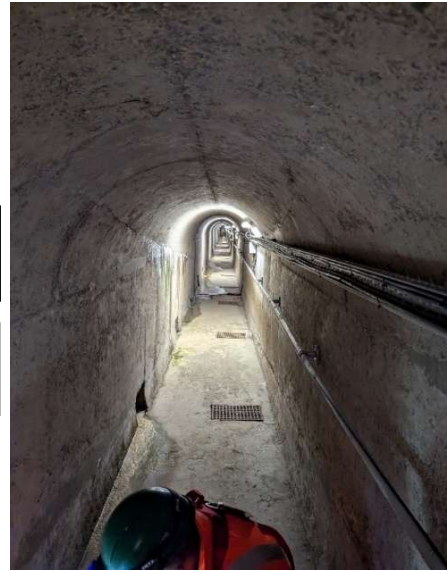
Figure 2. Photograph taken within the eastern drainage gallery
