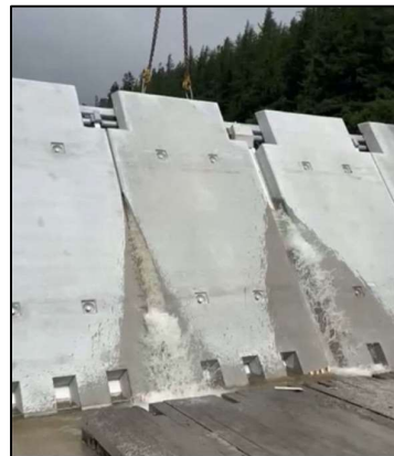
Figure 17. Commissioning the gates: photograph following a small movement away from the supports
