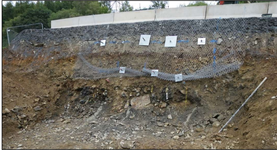
Figure 10. Soil nail trial panel
