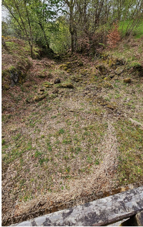
Figure 3. Main Spillway Channel
