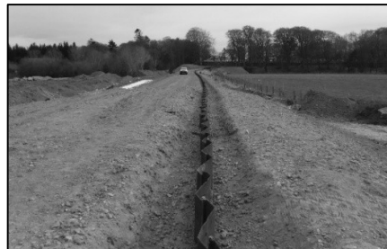
Figure 7. Completed partial cut off
