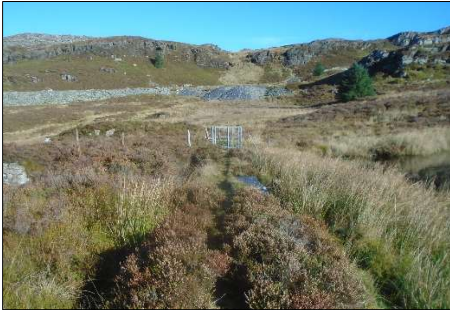
Figure 2. Dam crest viewed from the left abutment, taken during the 2022 Section 10 Inspection
