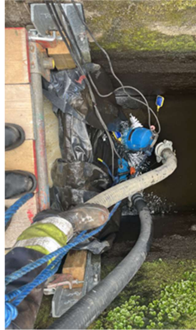
Figure 14: Installed Downstream Cofferdam with Pumps
