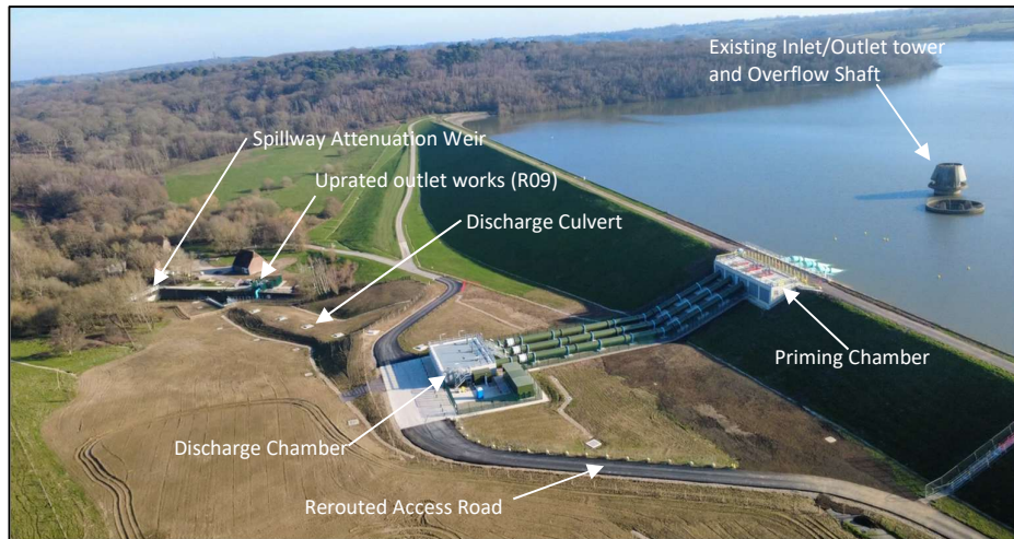
Figure 4: Aerial view of constructed drawdown scheme
