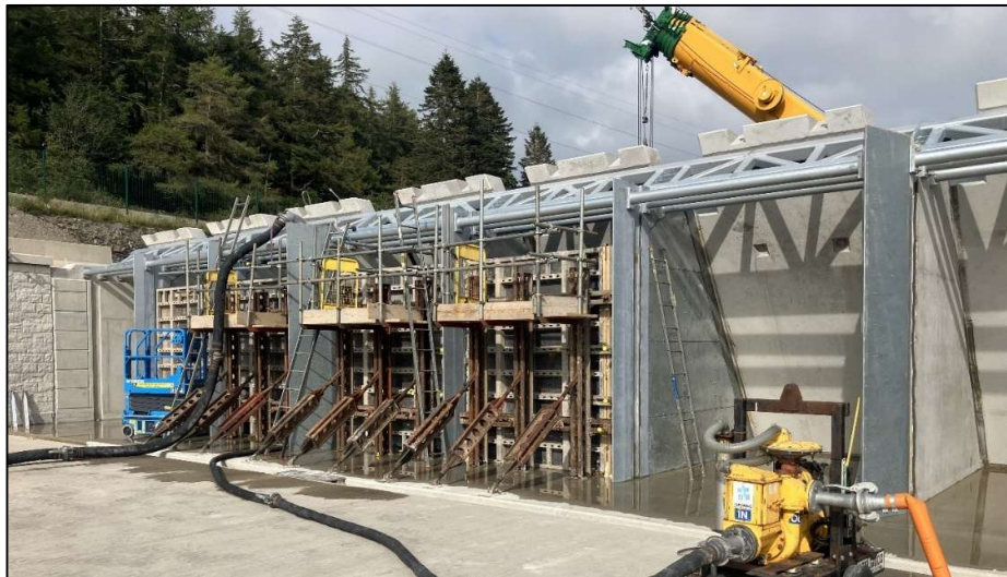
Figure 14. Tipping gates viewed from upstream during commissioning
