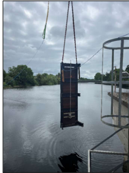
Figure 9: Photo of the Limpet Cofferdam being Lifted into Position for the Diving Contractor
