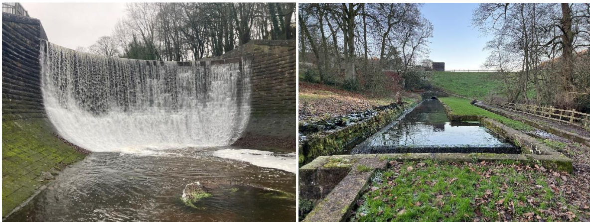
Figure 2 Spillway in flood (normally dry) and discharge flow measurement pond looking upstream at right half of dam
