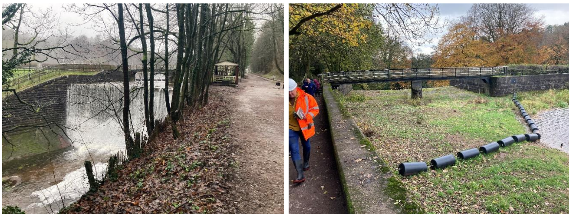
Figure 4 Rudyard Reservoir – spillway from left abutment with narrow gauge railway along the eastern bank, and spillway from upstream with floating boom to prevent anchored yachts from blocking the spillway during a storm (safety measure)
