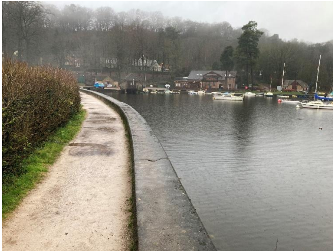
Figure 1 Dam crest – looking west
