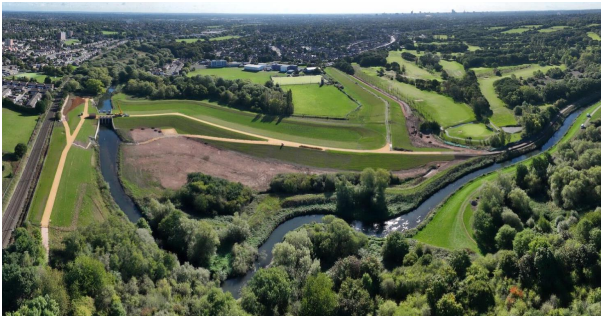
Figure 1 Drone view of completed dam
