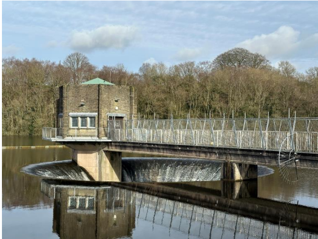
Figure 1 Tittesworth Reservoir Overflow
