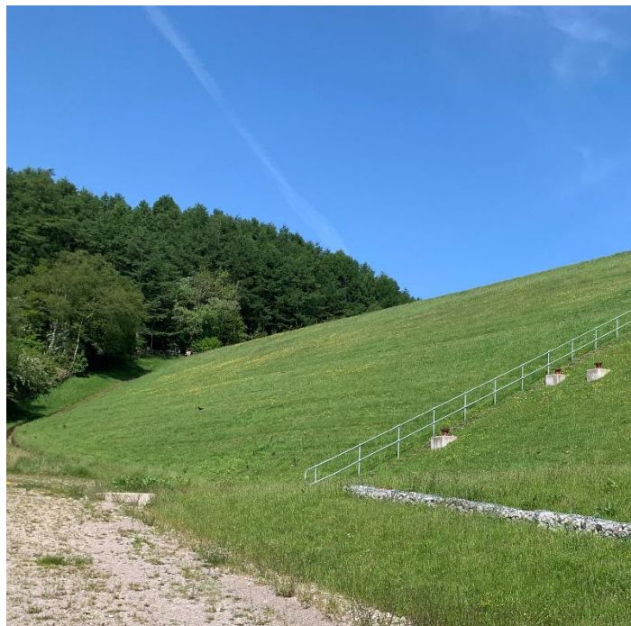
Figure 2 Tittesworth Reservoir Downstream Embankment
