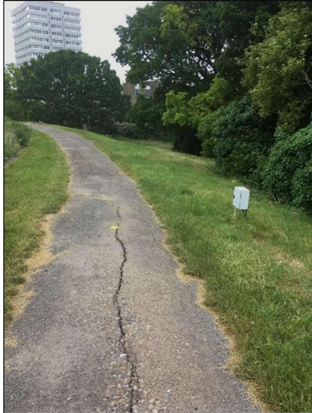
**Figure 2.** North-eastern portion of the embankment with shrinkage of clay in summer creating cracks in the crest path, looking north-east.
