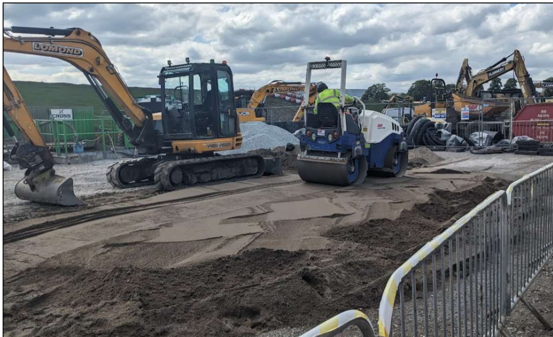
Figure 5. Fine Filter Compaction Trial
