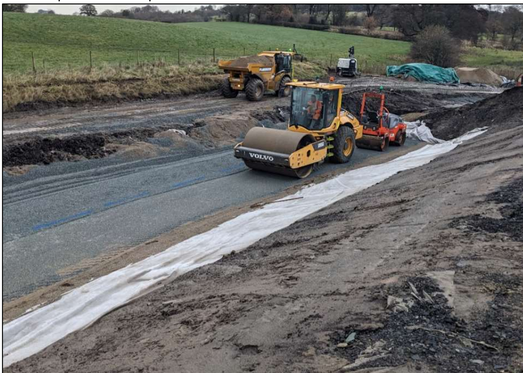
Figure 6. Compaction of coarse filter
