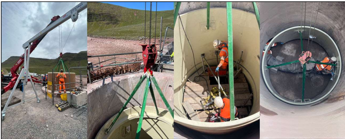
Figure 6. Installation of GRP Lining
