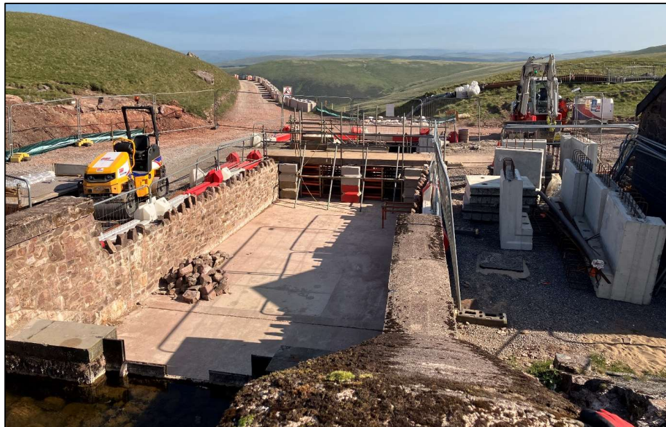
Figure 8. Spillway construction and lining
