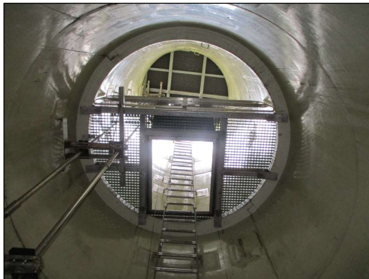
Figure 9. GRP Lining Installed
