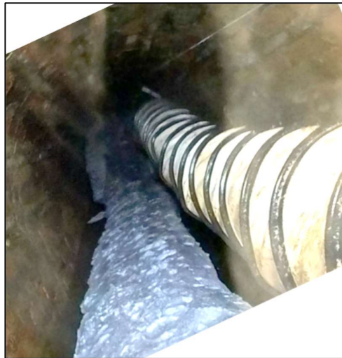
Figure 10. Expanding geopolymer foam in the adit
