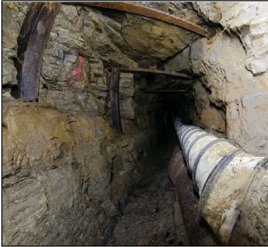
Figure 8. Adit view before start of drilling.
