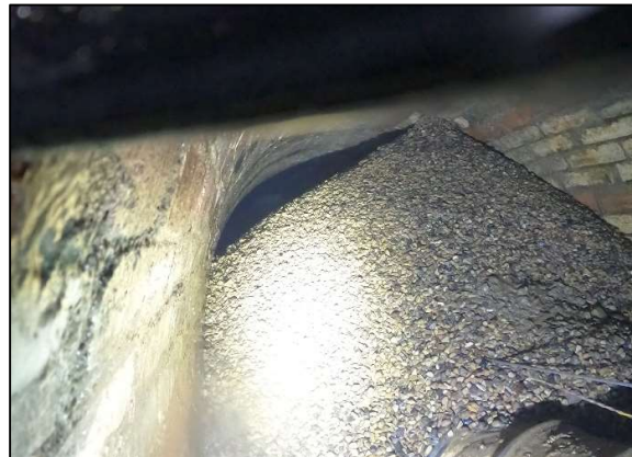
Figure 7. Post injection view of the mound with foam just visible beyond the gap.
