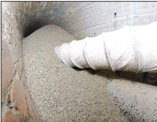
Figure 6. View of the pea gravel mound.
