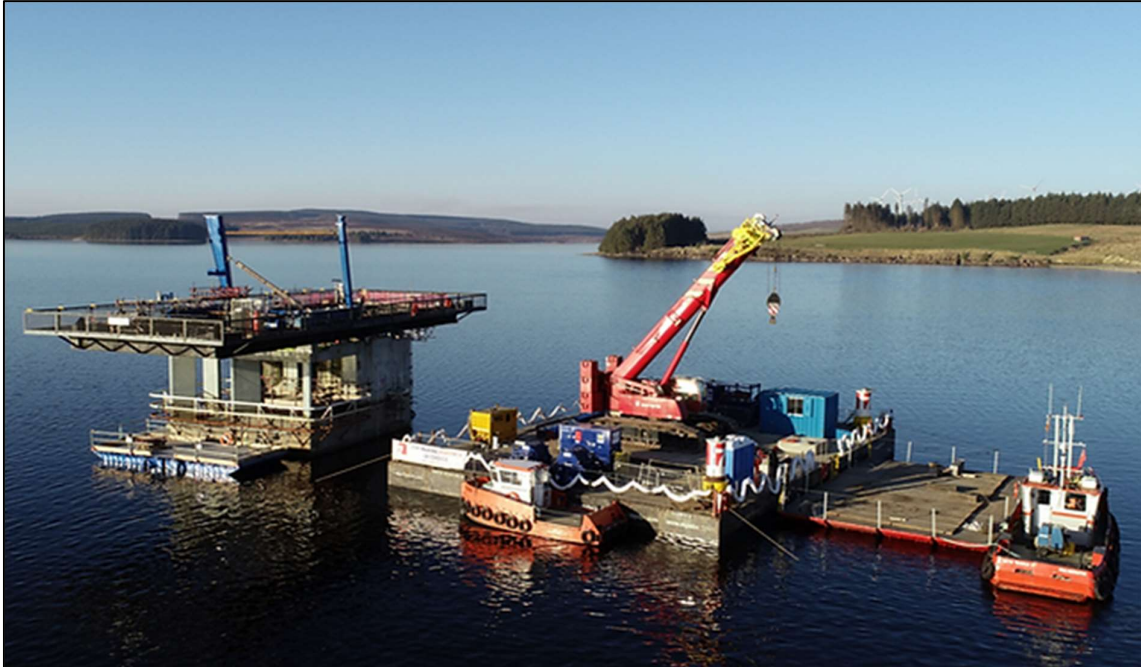
Figure 3. Pontoon in position and crane replaced (MMB)
