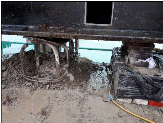
Figure 1. Hydraulic jack supporting crane during plinth replacement (MMB)
