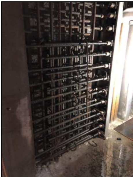
Figure 9. Completed reinforcement assembly prior to concrete profiling installation (MMB)
