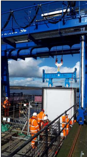
Figure 5. New Scour Bulkhead being lowered into position (MMB)
