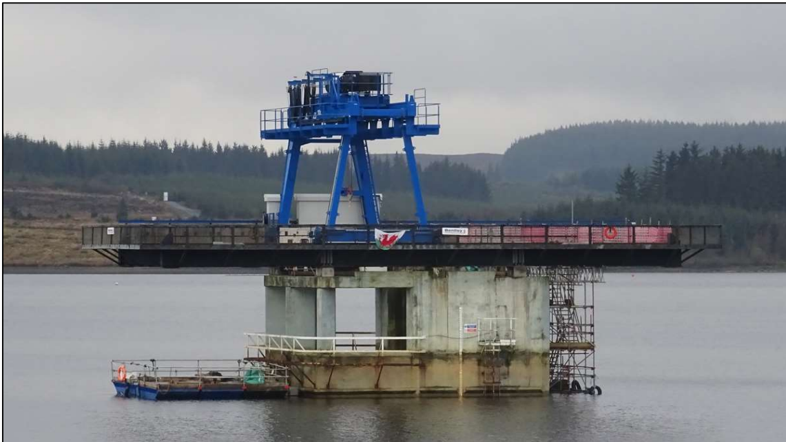
Figure 4. Completed crane installation (ARUP)
