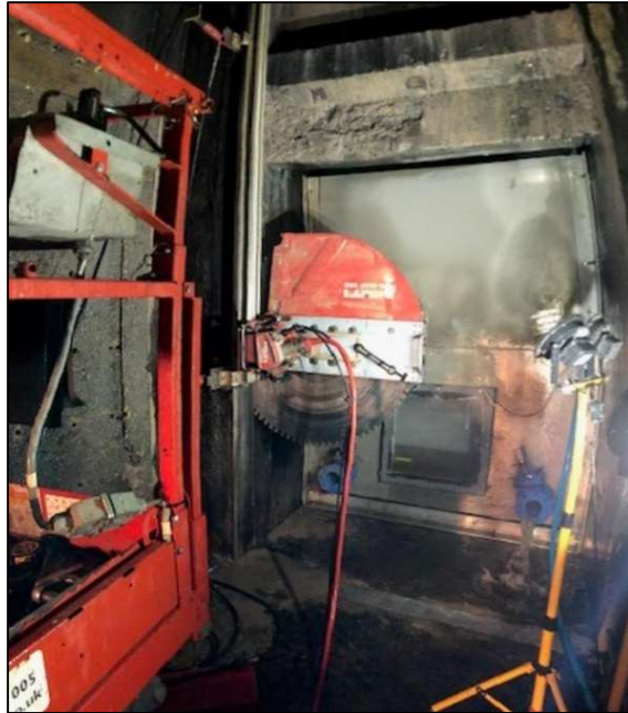
Figure 8. Installation of primary scour gate
