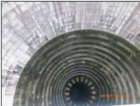
Figure 2. Bellmouth view from footbridge
