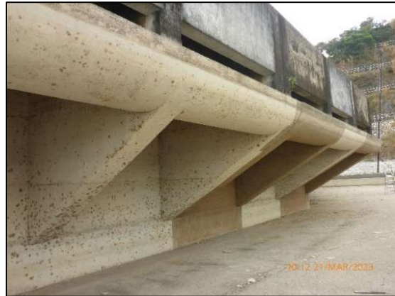
Figure 3. Siphon inspection with reservoir drawn down
