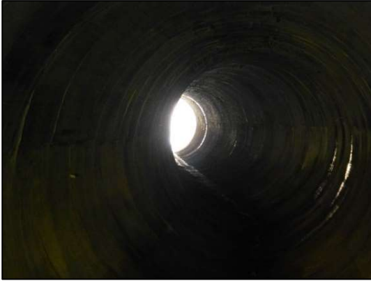
Figure 4. View from the base of the drop shaft
