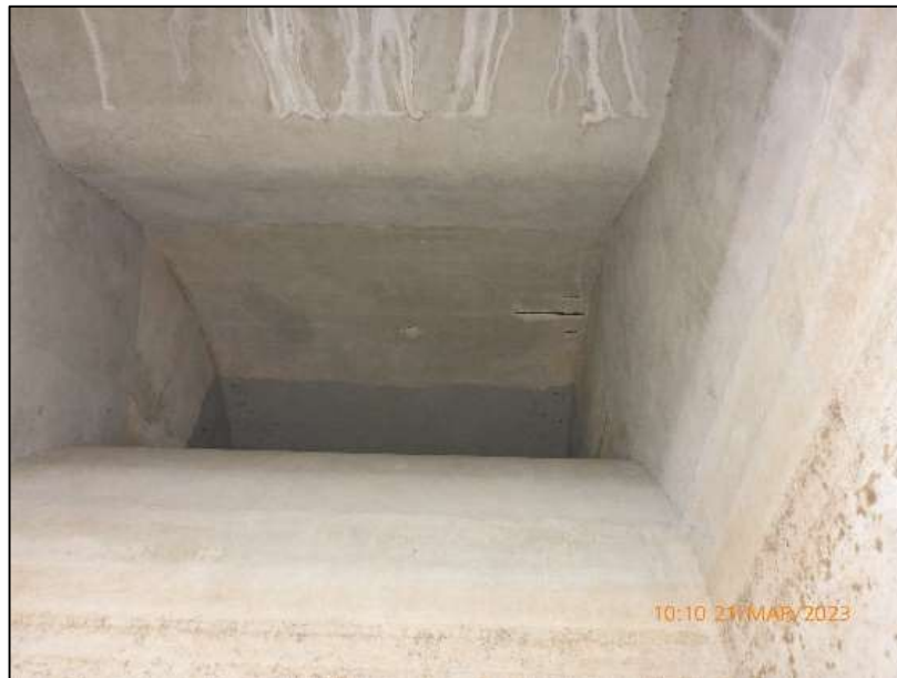
Figure 6. Siphon internal structure, view from downstream end of siphon.
