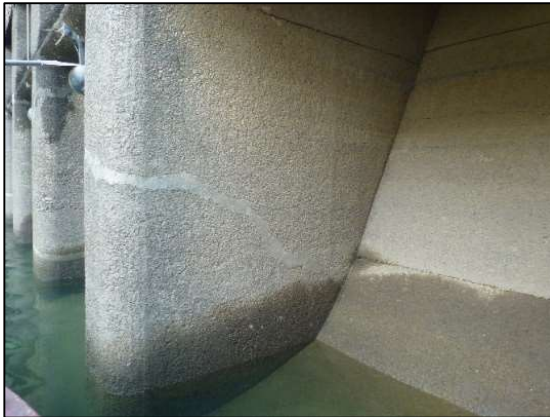
Figure 2. Siphon inlet inspection from a boat
