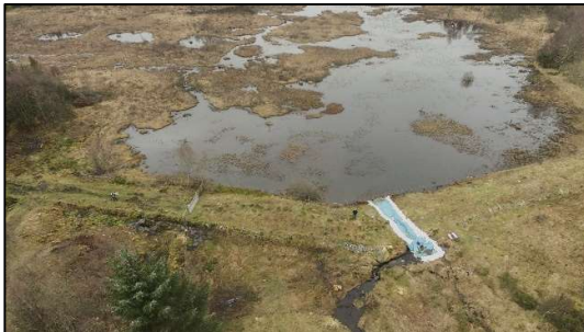
Figure 1. Temporary repairs at Tynmynydd.
