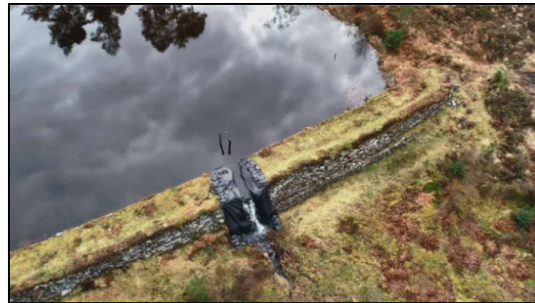
Figure 2. Temporary repairs at Pandora.
