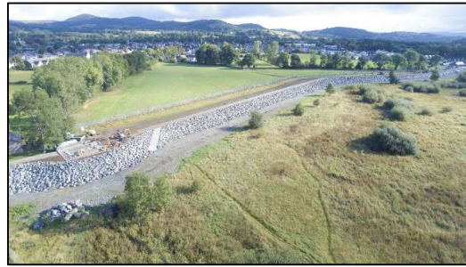
Figure 8. Llyn Tegid Overtopping embankment using reinforced grass.
