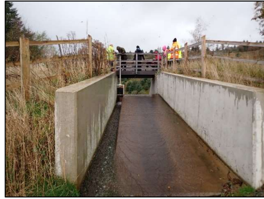
Figure 14. Bwlch, reinforced concrete spillway including drawoff.
