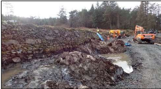
Figure 15. Pandora rock foundation.
