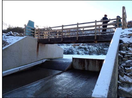
Figure 5. Llyn Llewelyn RC multistage weir, incorporating drawoff.
