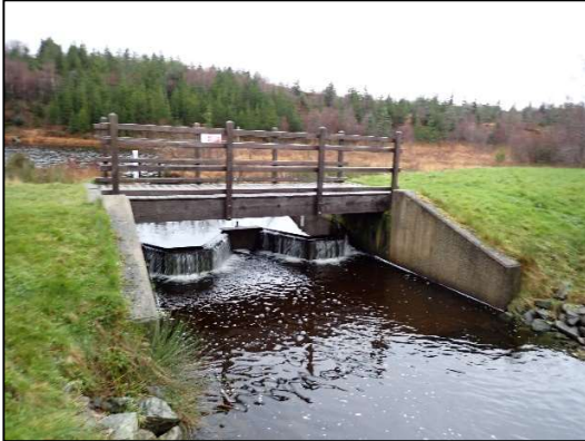
Figure 4. Llyn Goddionduon RC Labyrinth weir incorporating drawoff.
