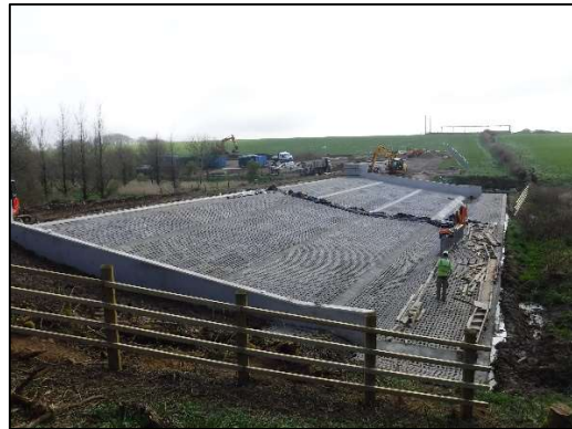
Figure 10. Pont y Cerbyd, Armorflex.
