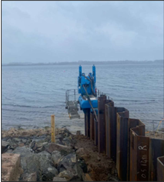
Figure 6. Installation of sheet piles using silent press (upstream)
