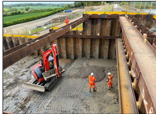
Figure 9. Blinding of Crest Chamber
