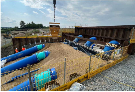
Figure 8. Backfilling siphon pipes downstream of Crest Chamber
