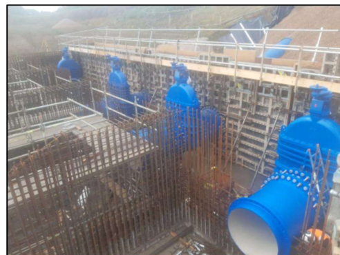
Figure 12. Construction of Outlet Chamber with outlet valves
