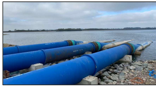
Figure 7. Installation of siphon upstream legs
