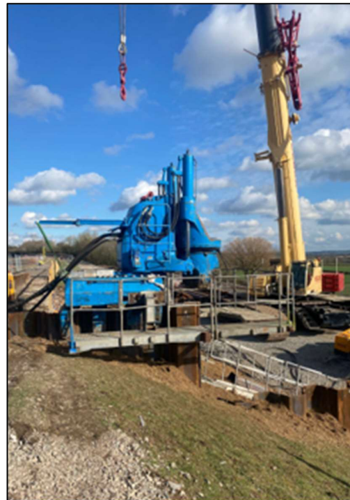
Figure 5. Installation of sheet piles using silent press (downstream)
