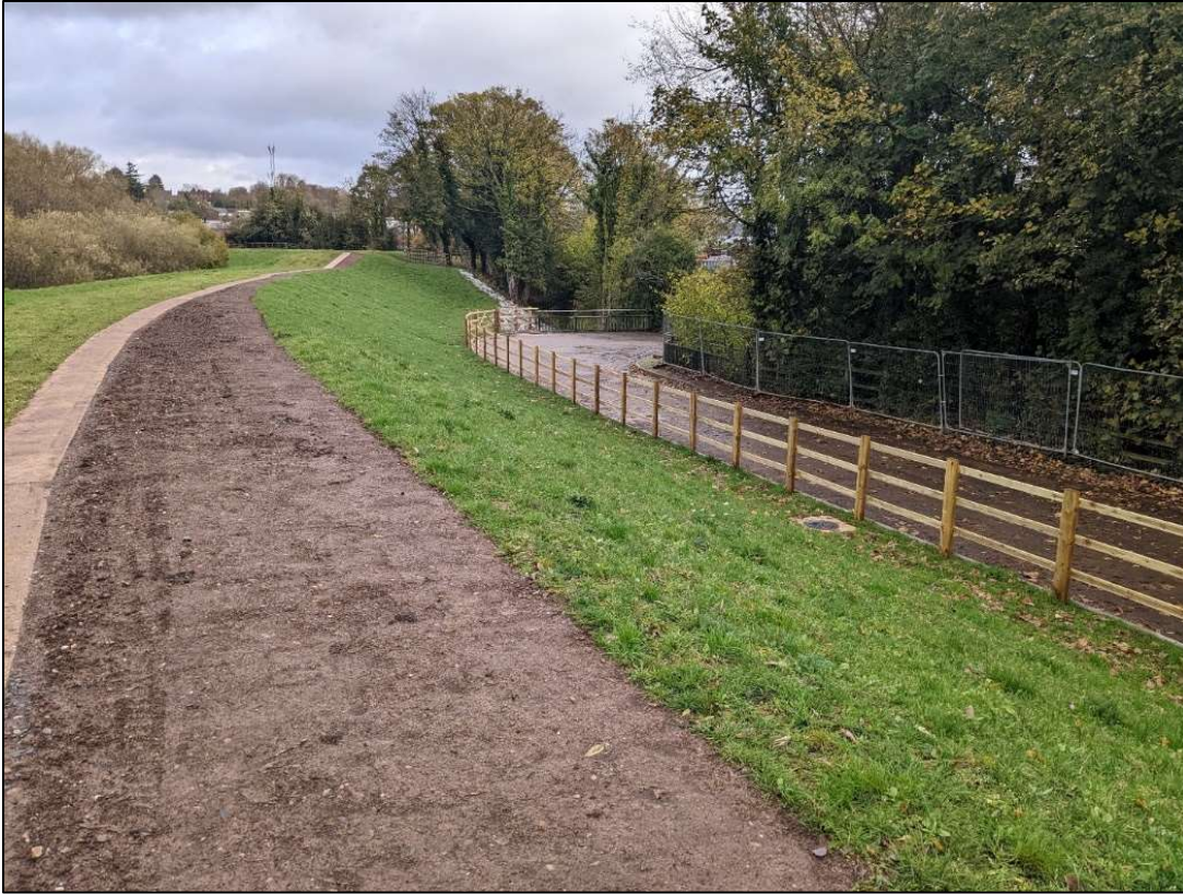
Figure 6. Completed spillway with turf installed
