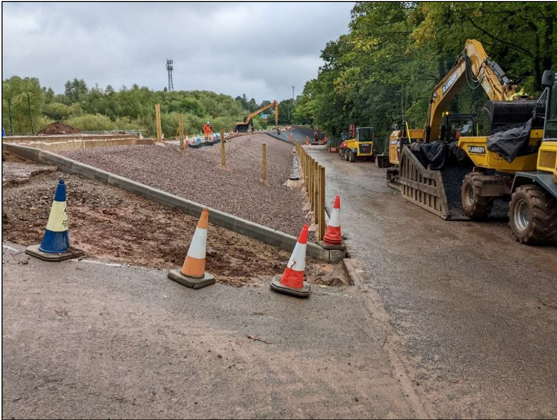
Figure 4. Placing OSA (dumper being loaded at downstream toe)
