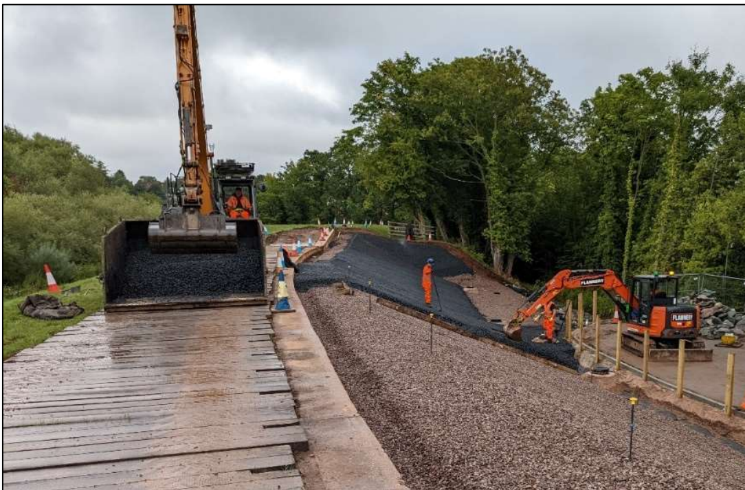
Figure 5. Placing OSA (long reach excavator taking OSA from skip on crest)
