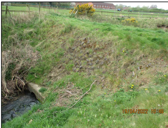
Figure 2. Access to Rase North throttle pipe
