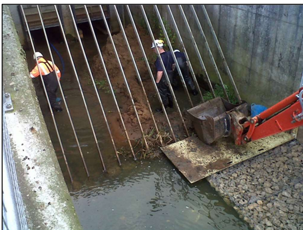
Figure 4. Rase South control structure being desilted (working in confined space)
