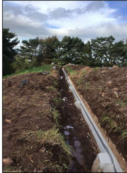
Figure 2. Repair of the roof / wall joint at Radyr SRV. (Courtesy of DCWW).
