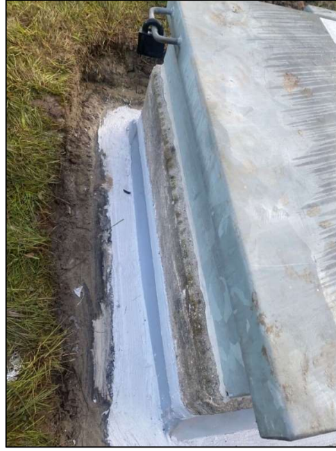
Figure 6. Repairs around a roof hatch at Tongwynlais No.2. (Courtesy of DCWW).
