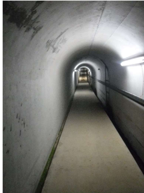
Figure 3. Photograph of drainage gallery
