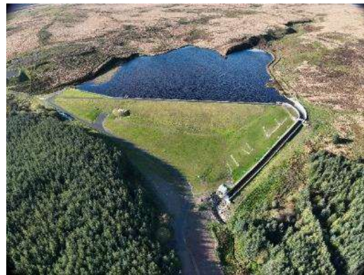
Figure 9. Works complete (DCWW)
