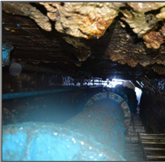
Figure 4. ‘Dry’ well tower access (looking up) prior to works (MMB)
