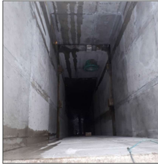
Figure 5. Lined fully ‘dry’ valve tower (looking down) (MMB)
