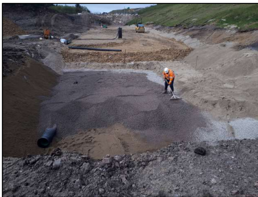
Figure 8. Installation of toe drain and filters (MMB)
