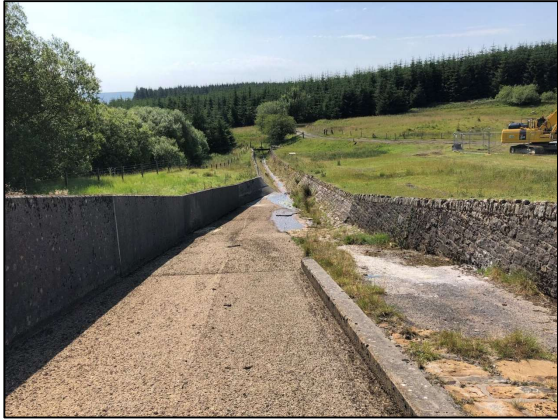
Figure 10. Previous composite spillway (MMB)
