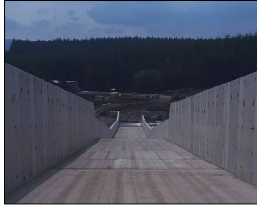
Figure 11. New reinforced concrete spillway (MMB)
