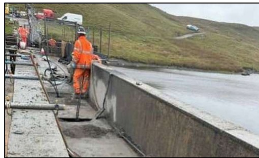
Figure 14. Anchors being installed on the abutment walls (MMB)
