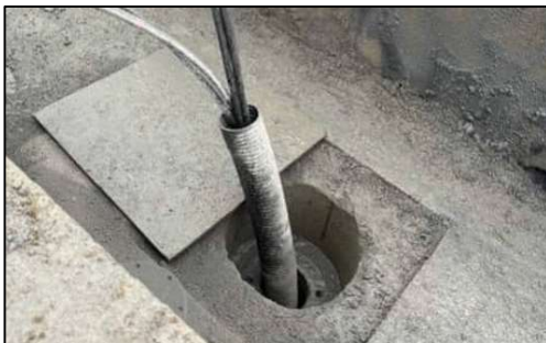
Figure 13. Anchors being installed on the abutment walls (MMB)
