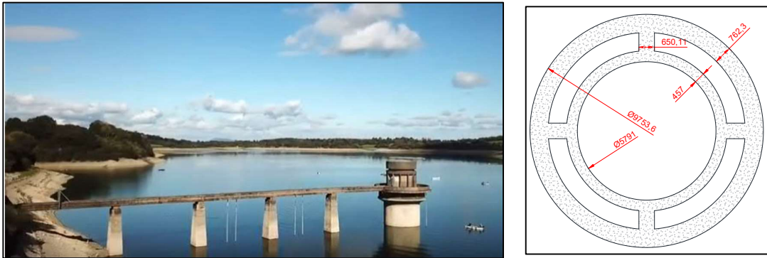
Figure 1. Llandefydd water draw-off tower and access footbridge
