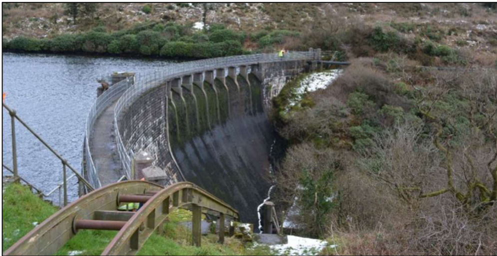
Figure 5. Rosebush Dam (MMB)
