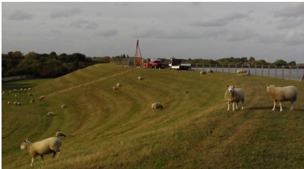
Figure 1. Cable percussion borehole through Island Barn embankment dam.
