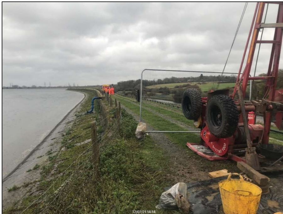
Figure 3. Cable percussion borehole through KGV embankment dam (provided by MWHT).
