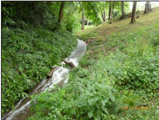
Figure 5. Original spillway channel
