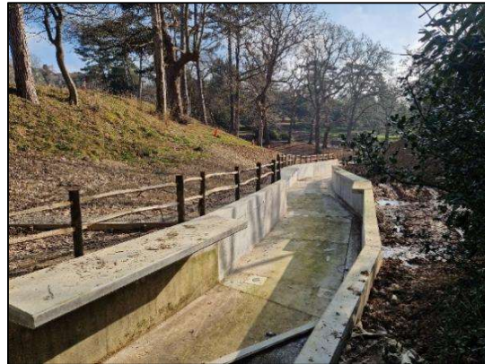
Figure 6. New spillway channel
