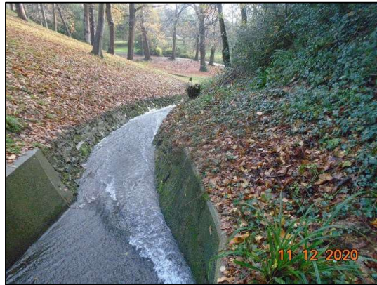
Figure 6. View of transition to original masonry channel
