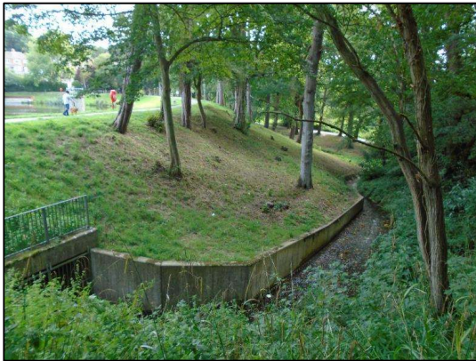
Figure 5. View of 1985 spillway channel section (from right abutment)
