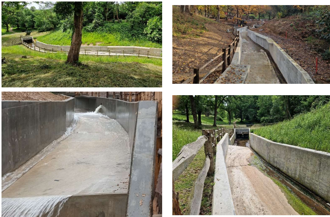
Figure 15. Finished spillway channel and stilling basin
