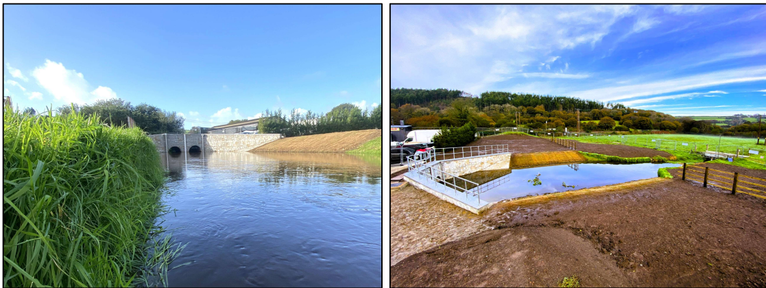
Figure 4. Images of the completed St Blazey FSR discontinuance
