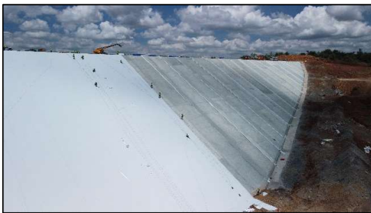
Figure 13. Installation of geomembrane on porous concrete at lower dams
