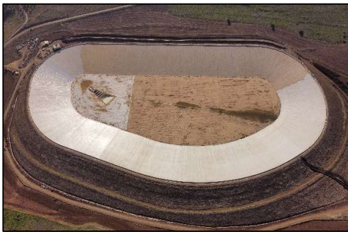
Figure 5. Kokhav Hayarden upper reservoirs' liner being completed
