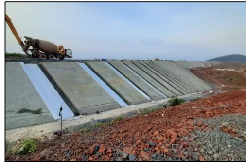
Figure 12. Geomembrane anchor bands embedded in trenches
