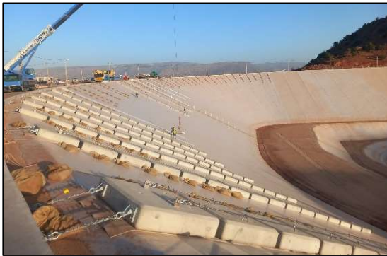
Figure 9. Some additional ballast at Abdelmoumen upper reservoir
