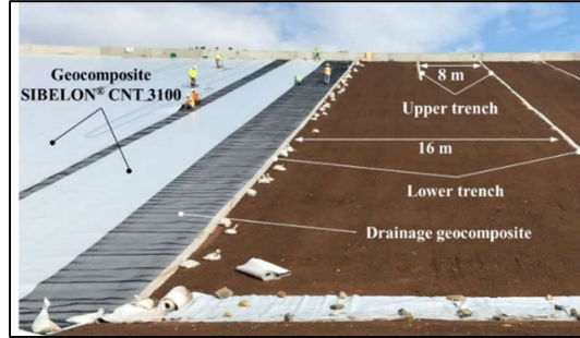
Figure 4. Components of the waterproofing system
