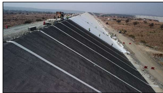
Figure 14. Installation of geomembrane on synthetic drain at upper dam
