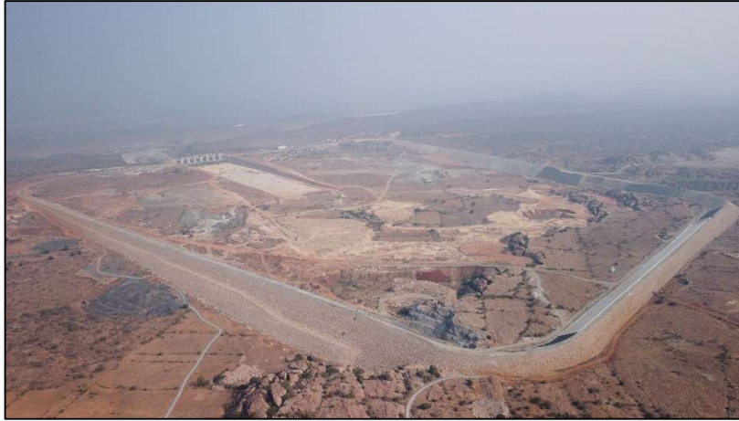
Figure 15. Pinnapuram pumped storage scheme: upper reservoir
