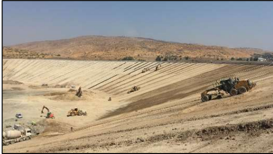
Figure 3. Preparation of subgrade and anchor trenches at Kokhav Hayarden
