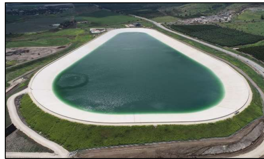
Figure 6. Kokhav Hayarden lower reservoir impounding
