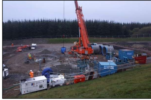
Figure 24. Shaft installation
