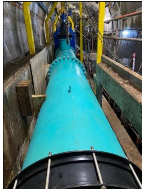
Figure 8. New pipework installation
