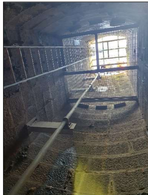
Figure 22. Access within valve tower
