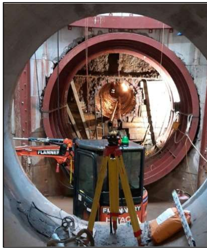
Figure 25. Tunnel installation pre-infilling
