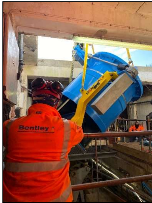
Figure 10. New valve installation
