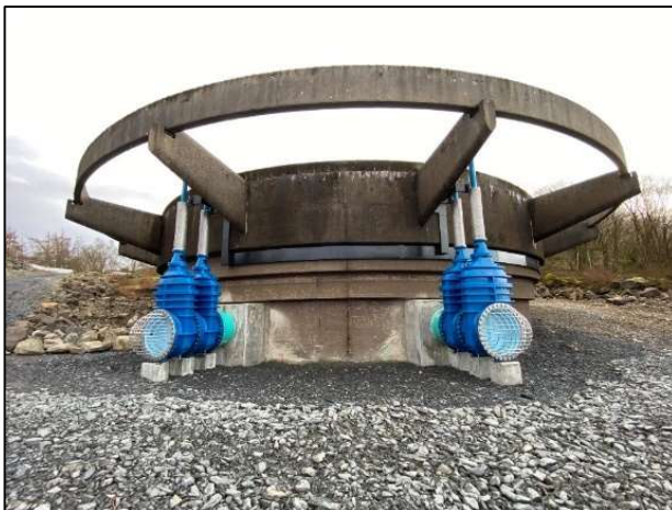
Figure 13. New drawdown facility
