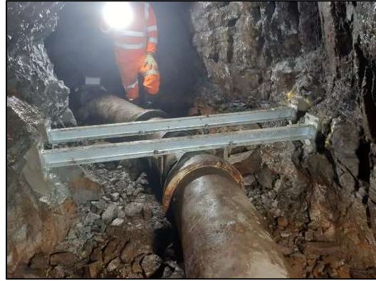
Figure 28. Thrust restraints
