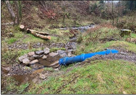
Figure 27. New scour outlet
