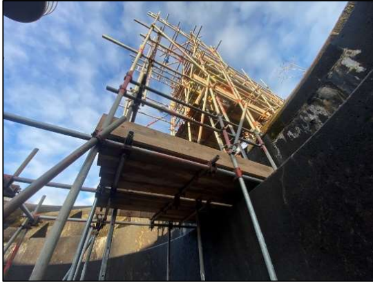
Figure 11. Scaffold installation
