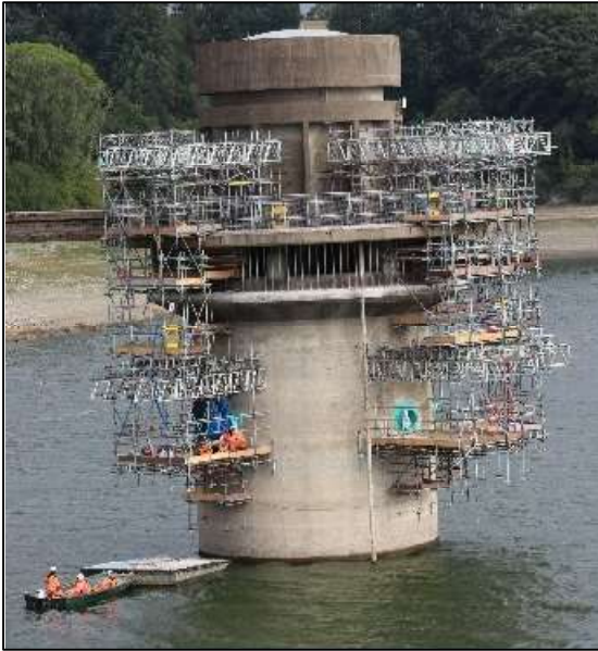
Figure 15. Scaffold arrangement
