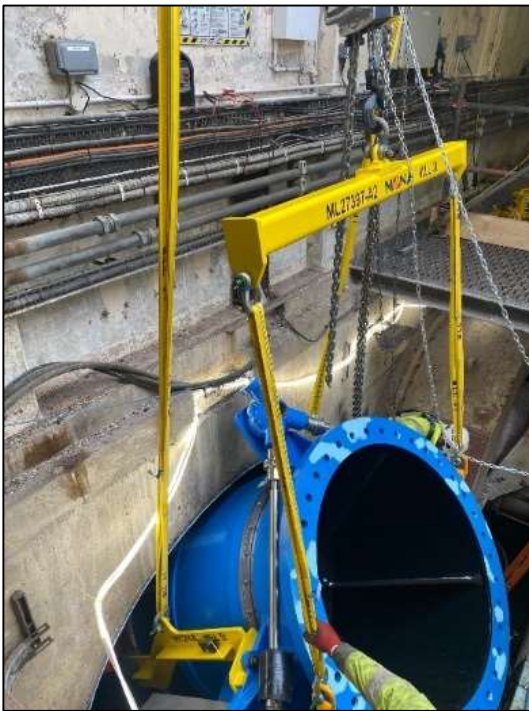
Figure 9. New valve installation
