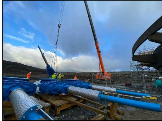
Figure 12. New valves and crane
