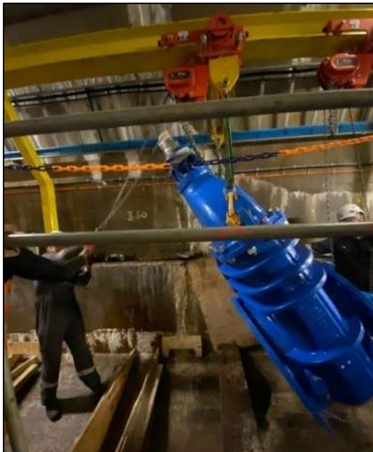
Figure 7. New valve installation
