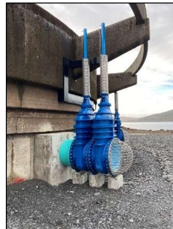
Figure 14. New drawdown facility
