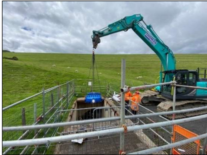
Figure 6. New valve being lowered being into tunnel
