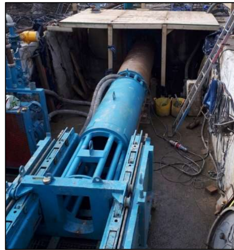
Figure 26. Micro-tunnelling scour main
