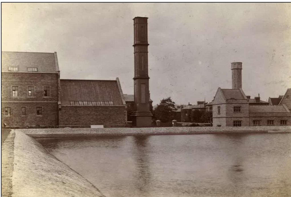
Figure 2. Reservoir conversion works in progress showing the original overflow shaft and reservoir lining.
