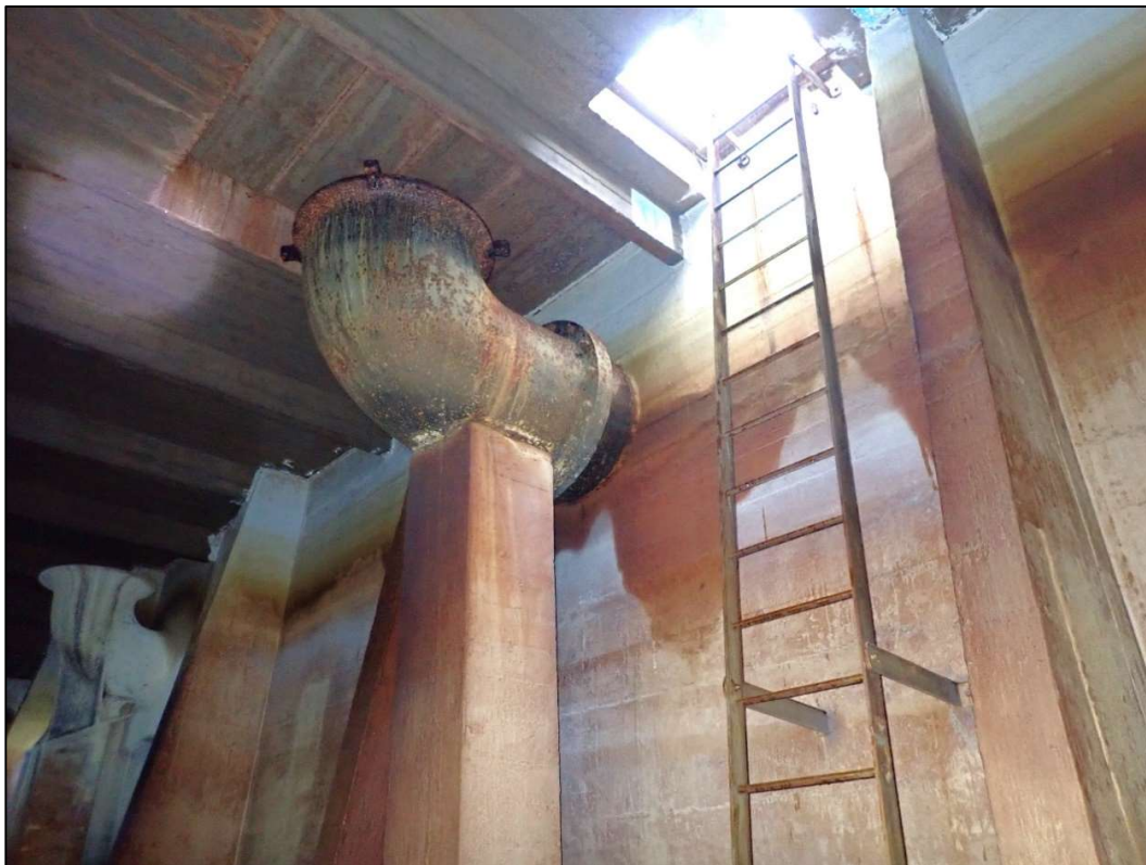
Figure 3. Southern wall and inlet pipework in 1915 (above) and 2023 (below)
