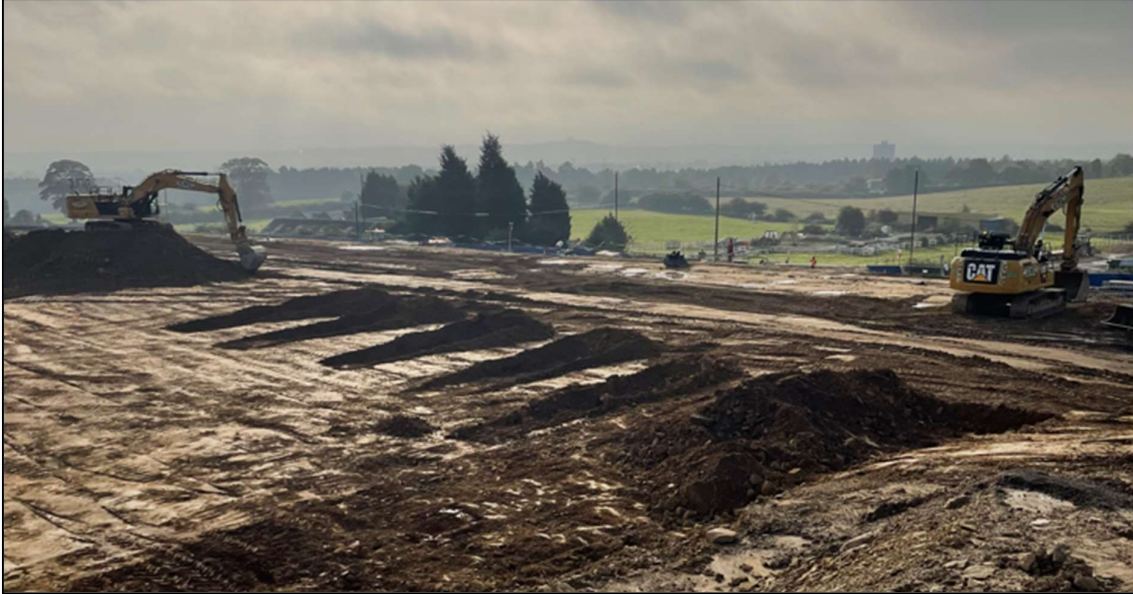
Figure 8: Transition from competent to weathered rock inspection trenches
