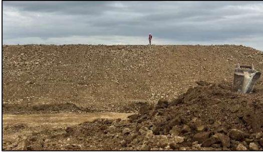
Figure 4 Constructed surcharge bund
