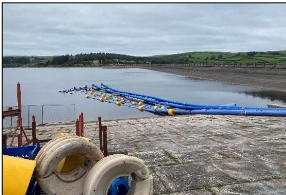
Figure 5. Usk Reservoir siphon and over pumping intakes
