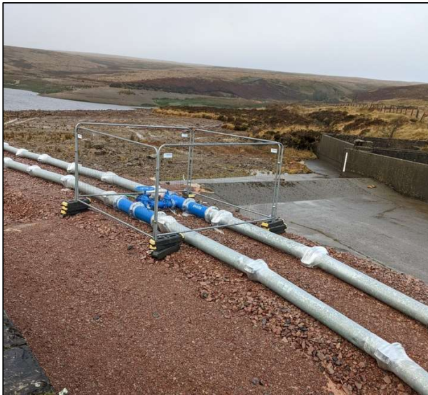
Figure 3. Upper Carno siphon priming point
