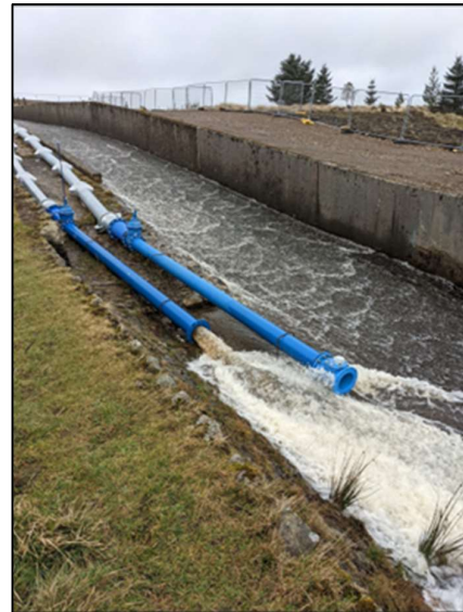
Figure 4. Upper Carno siphon discharge point. Note flows from By-wash channel
