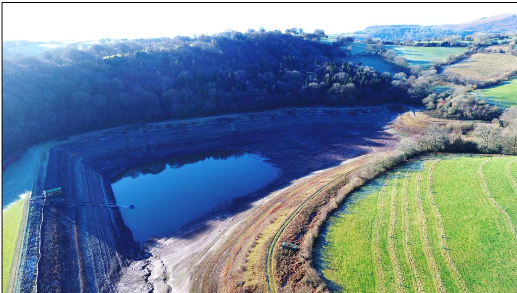
Figure 1. Pumping arrangement adjacent to Pant yr Eos dam. Right-hand bywash visible in the background
