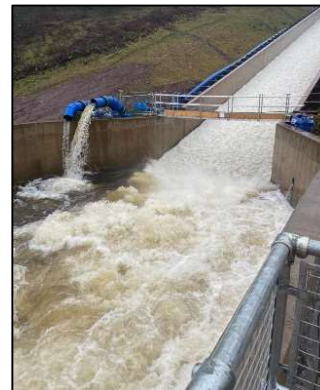
Figure 6. Usk Reservoir siphon outfall
