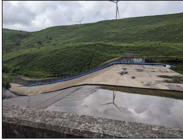
Figure 9. Castell Nos – Twin siphons installed
