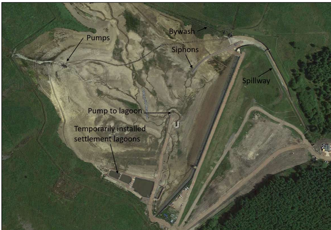
Figure 2. Upper Carno – Aerial image of Upper Carno drawn down with pumps and siphons shown to left hand side (Google Earth – modified)
