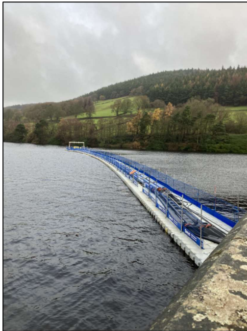
Figure 8. Gouthwaite Reservoir – Pumping pipework arrangement
