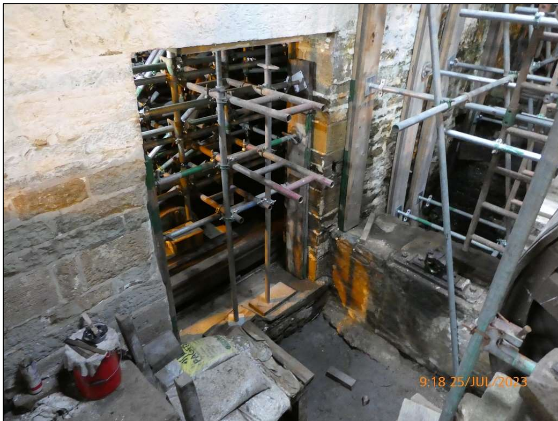
Figure 7. Scaffolding support to the walls of the 'Grinding Hull' building
