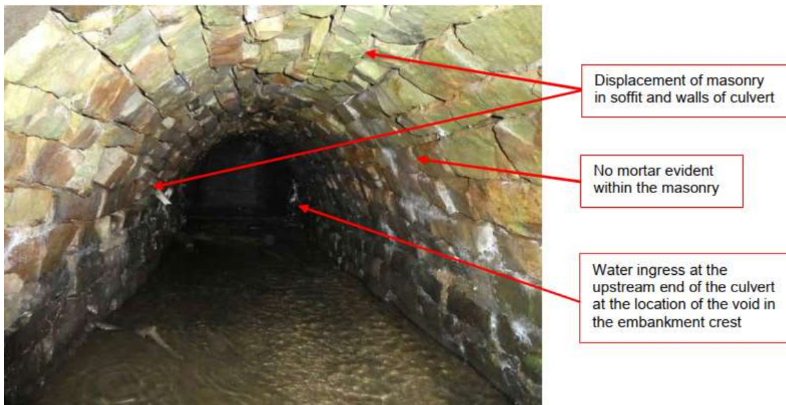
Figure 5. General condition of spillway culvert
