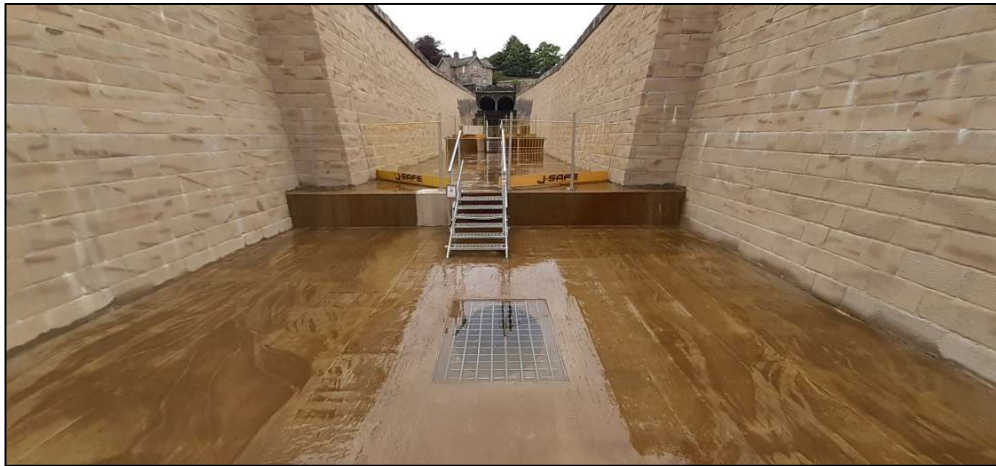
Figure 8. Siphon outlet in spillway invert
