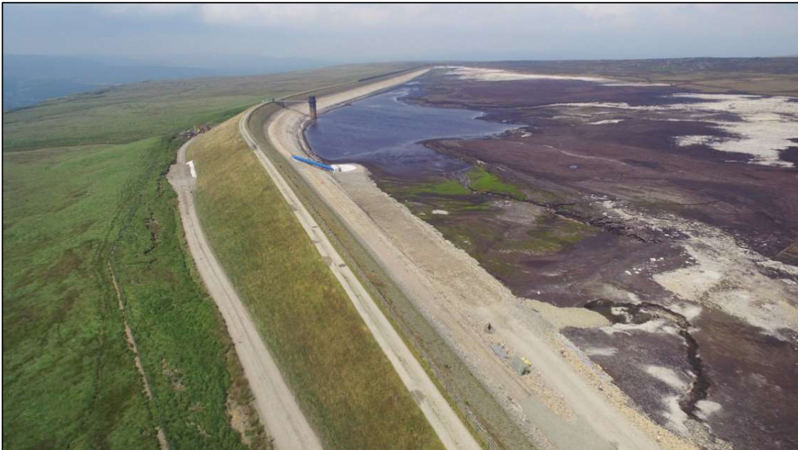
Figure 1. Warland Reservoir drawn down by 8m, and upstream pipe work installed
