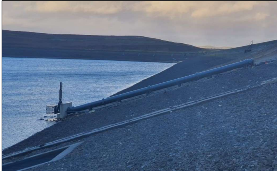
Figure 9. Upstream leg of siphon
