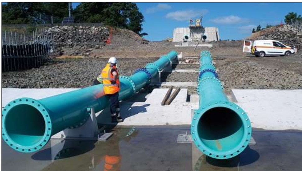
Figure 12. DN700 siphon pipework during installation
