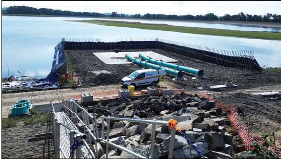
Figure 11. Siphon intake bay constructed within the cofferdam.
