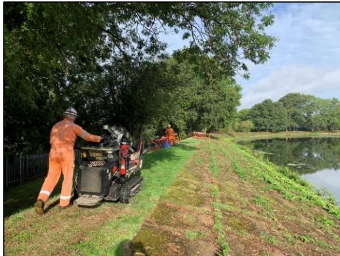
Figure 3. Small portable drilling rig on narrow crest
