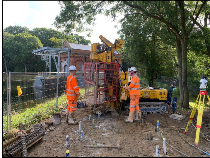
Figure 7. Drilling works on the crest
