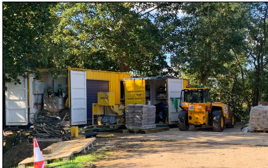
Figure 6. Site compound area for grouting equipment
