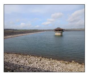
Carsington Reservoir is located 5 kilometres south west of Wirksworth, Derbyshire on the Henmore Brook. It is the ninth largest reservoir in England. The dam is 34.3m high, by 1200m long, and the reservoir has a capacity of 36,000,000m<sup>3</sup>. It is primarily pumped storage, used to supply Water Treatment Works in the Derbyshire area.
