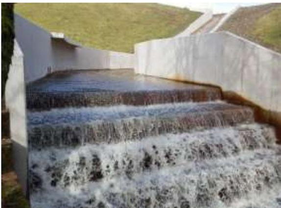
*Figure 4. New Spillway at Rhymney Bridge No2*
