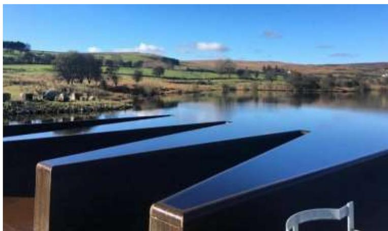
*Figures 1& 2. New Spillway and Labyrinth Weir at Shon Sheffrey Reservoir*
