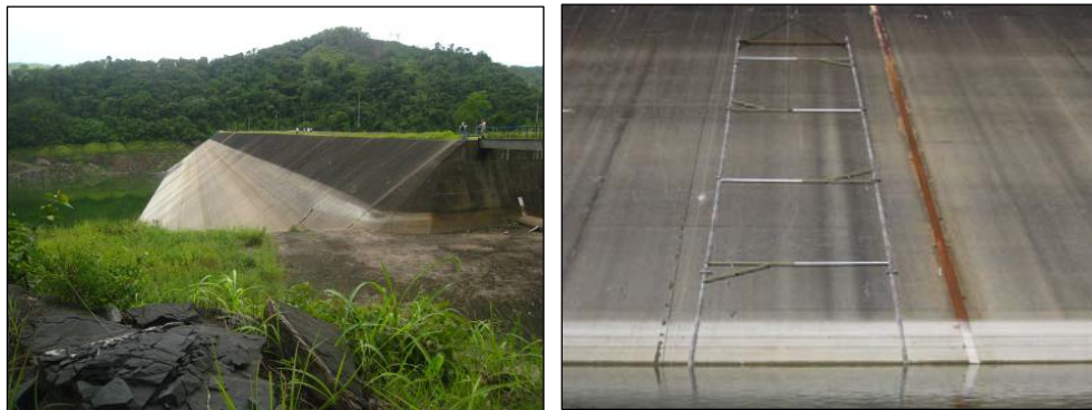
Figures 11 and 12. The vertical anchorage profiles being lowered in to the water
