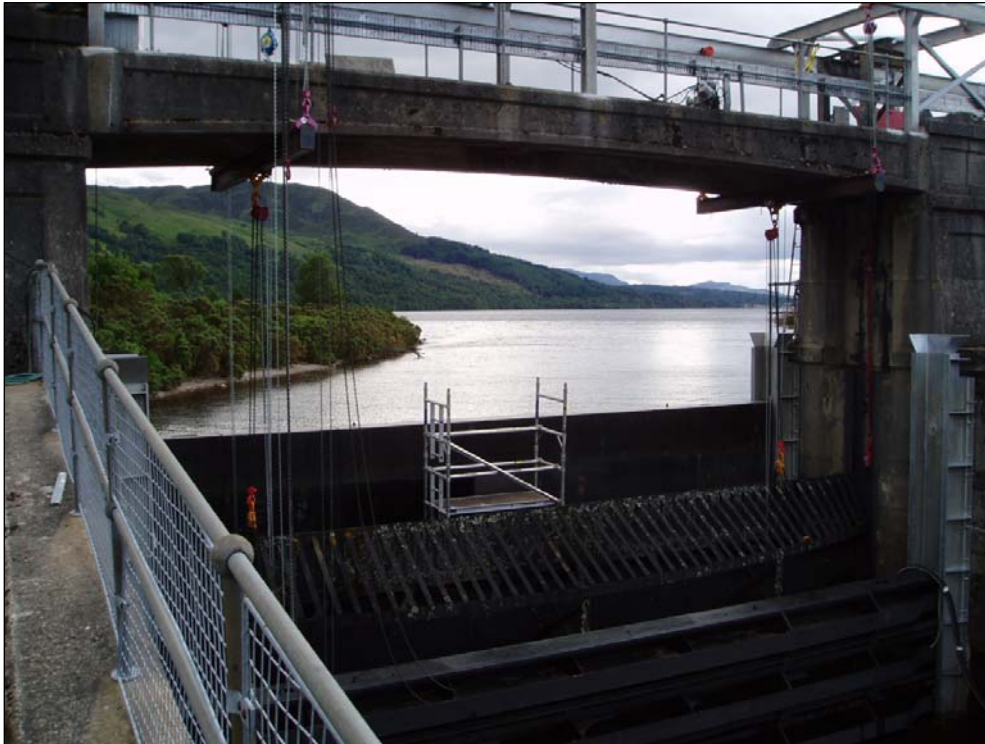
Figure 4. Photograph showing the stoplogs installed on site
