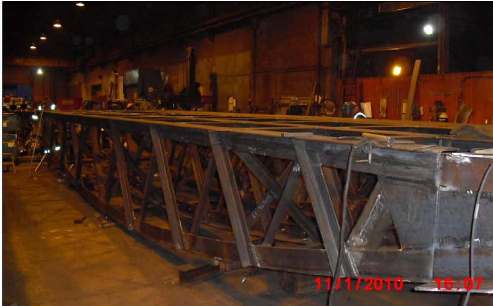
Figure 9. Photograph showing construction progress on gate #1
