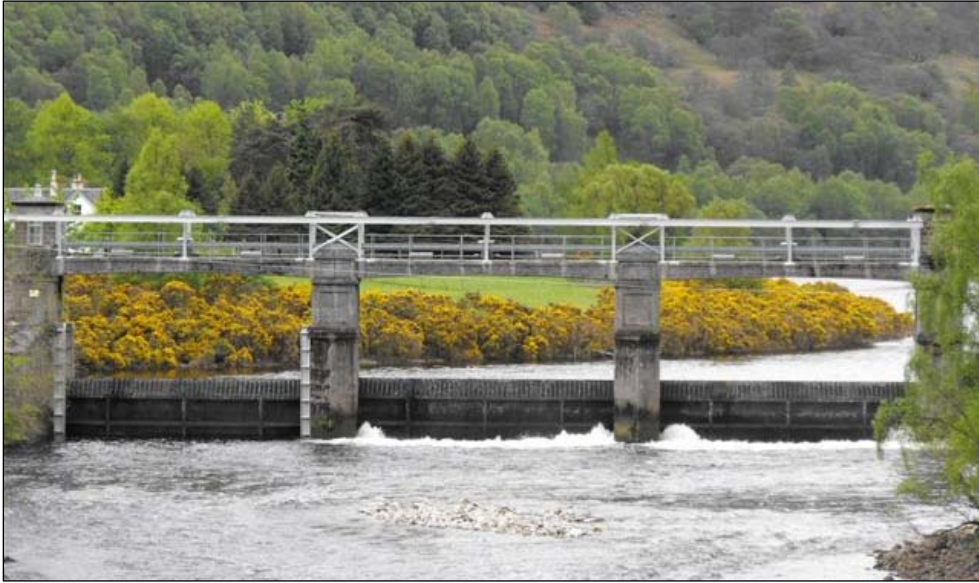
Figure 1. Photograph of Kinloch Rannoch Weir taken from downstream
