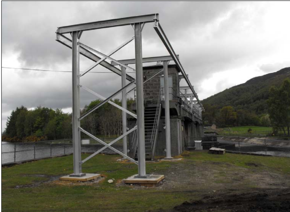
Figure 3. Photograph showing the bespoke stoplog installation frame
