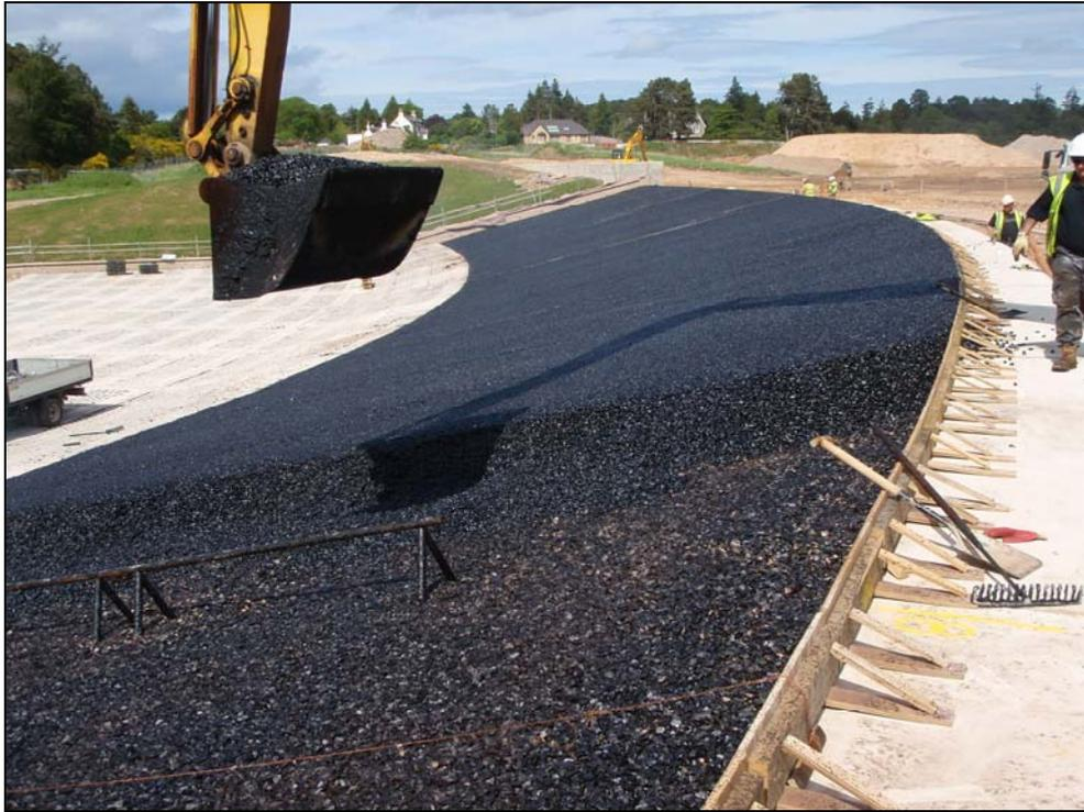
Figure 7 Laying open stone asphalt
