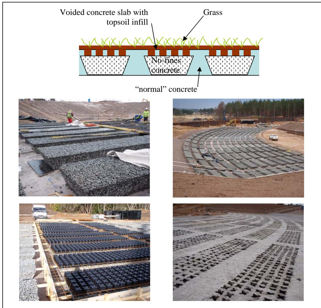
Figure 8. Voided concrete slab
