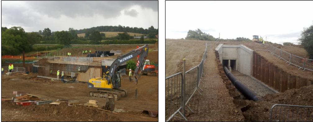
Figures 7 and 8. Inlet structure in construction and pipe through structure.
