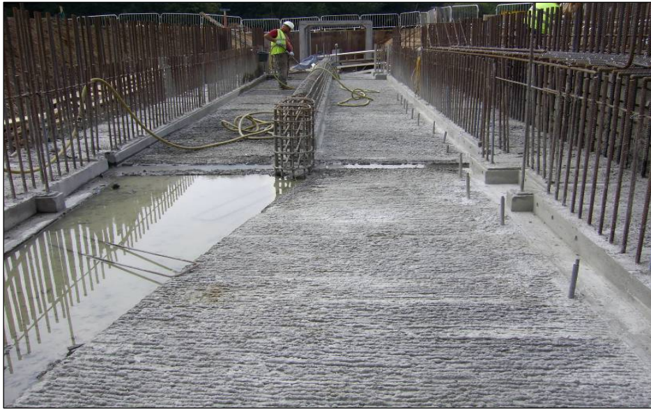
Figure 5. Textured bed at inlet achieved with a rake finish
