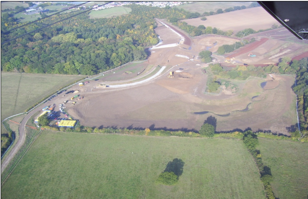
Figure 6. Aerial view of the reservoir under construction.
