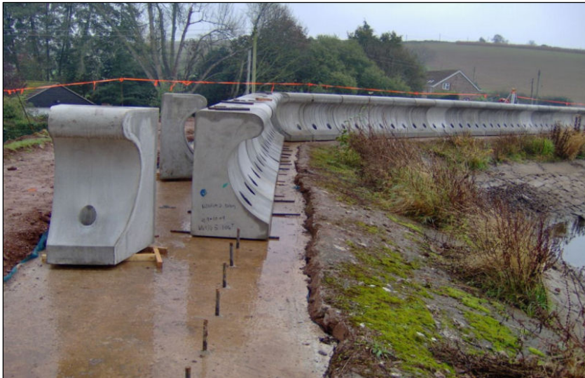
Photo 1 Construction of the new wewall
