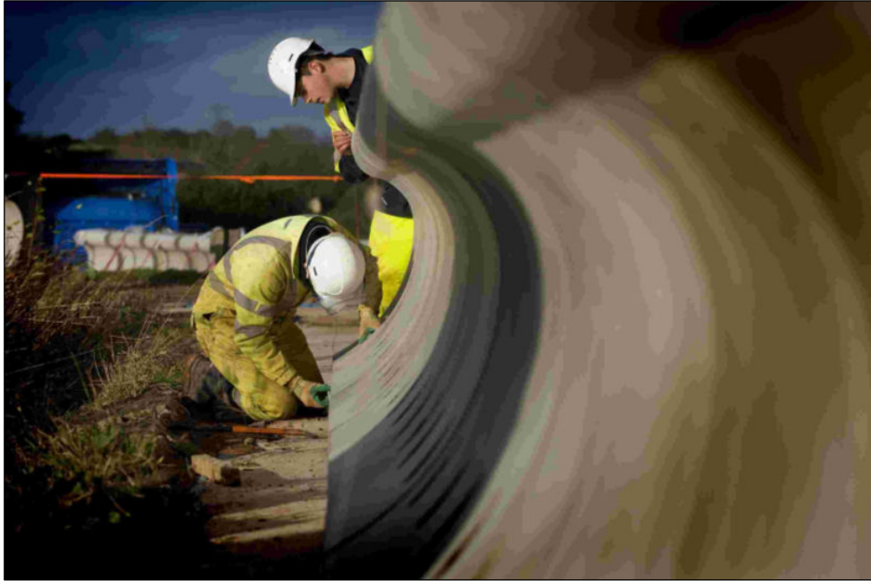
Photo 2 Levelling wavewall
