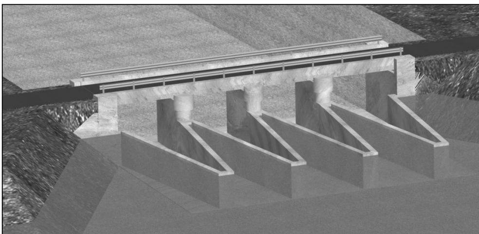
Figure 1. Proposed labyrinth weir and new access bridge
