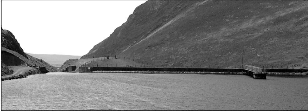
Figure 2. Craig-y-Pistyll dam in 2006, showing spillway via rock cutting at the left abutment
