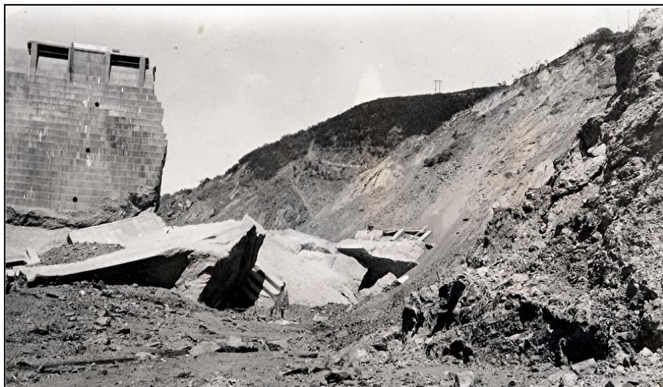
Figure 5. St. Francis Dam Left Abutment
