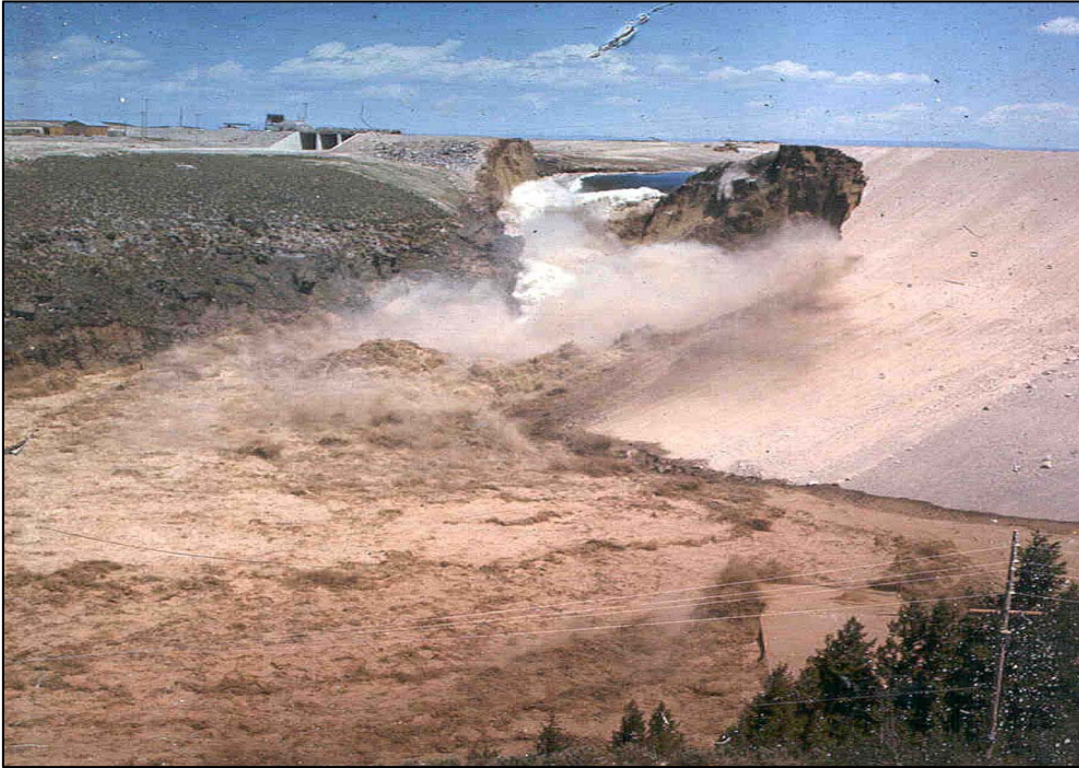
Figure 8. Teton Dam Minutes After Full Breach
