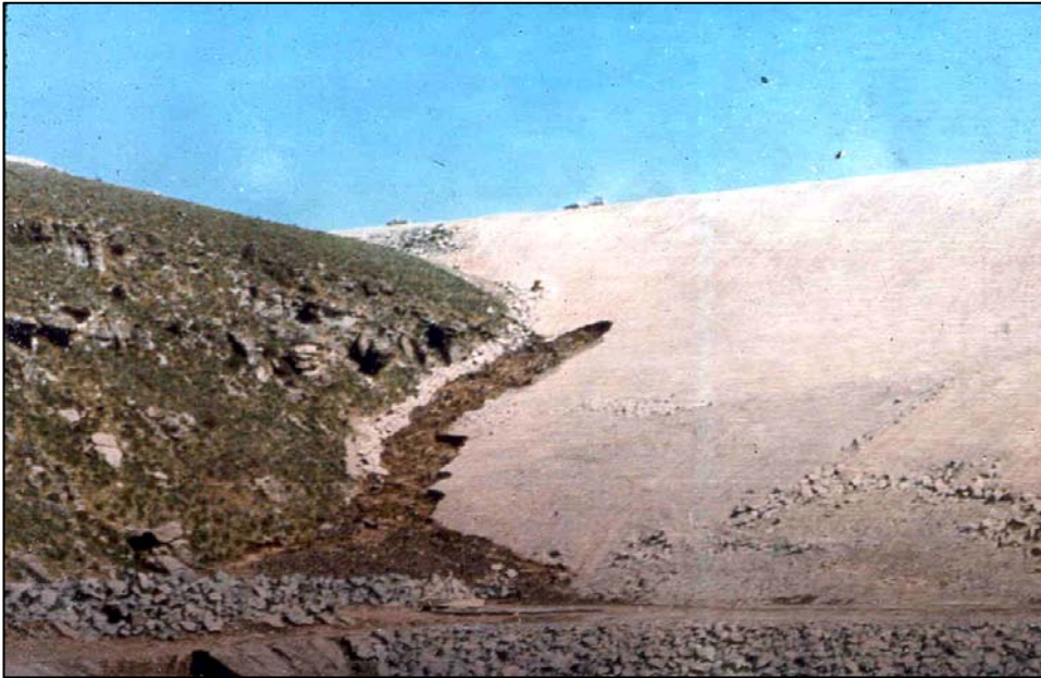
Figure 7. Right Abutment Seepage One Hour Before Failure
