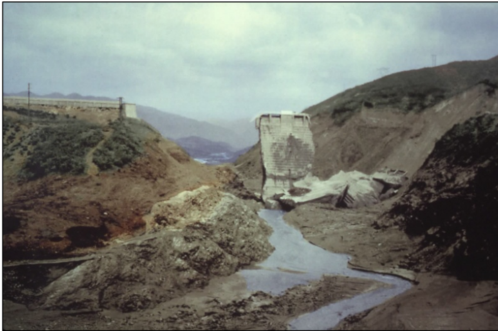
Figure 4. St. Francis Dam Immediately After Failure
