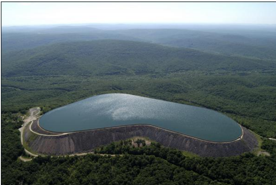
Figure 9. Taum Sauk Dam Before Failure
