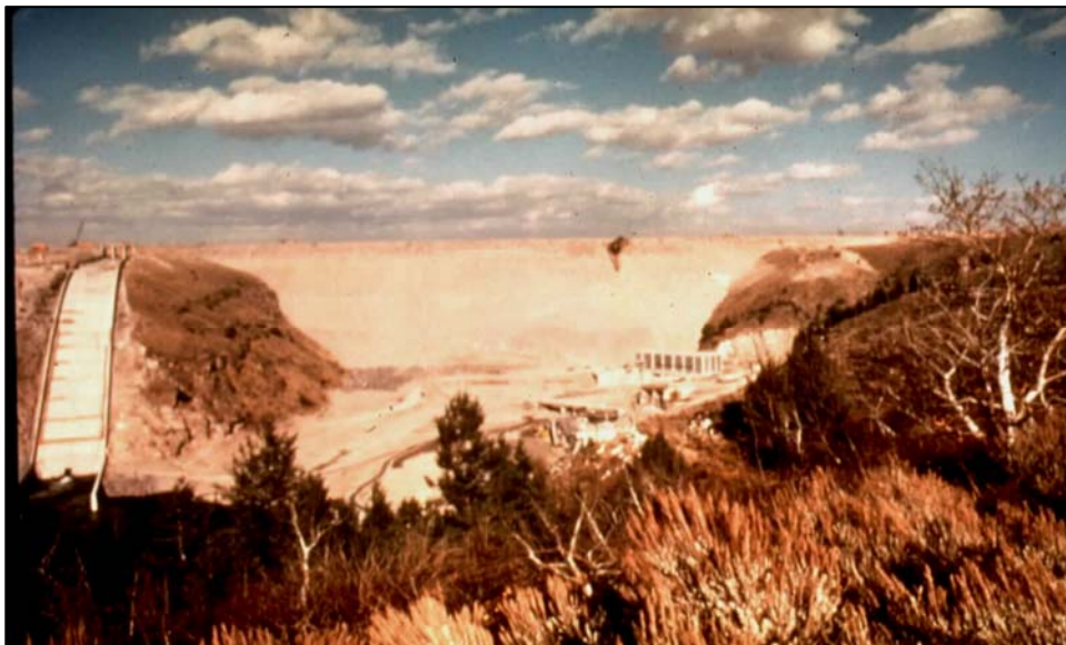
Figure 6. Teton Dam Days Before Failure
