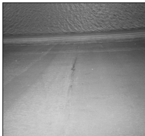
Figure 3. Day joint in Panel D47
