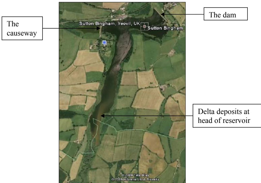
Figure 1. Aerial view of Sutton Bingham reservoir
