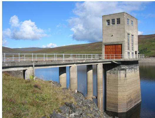
Figure 1: View of Errochty tower and access bridge
