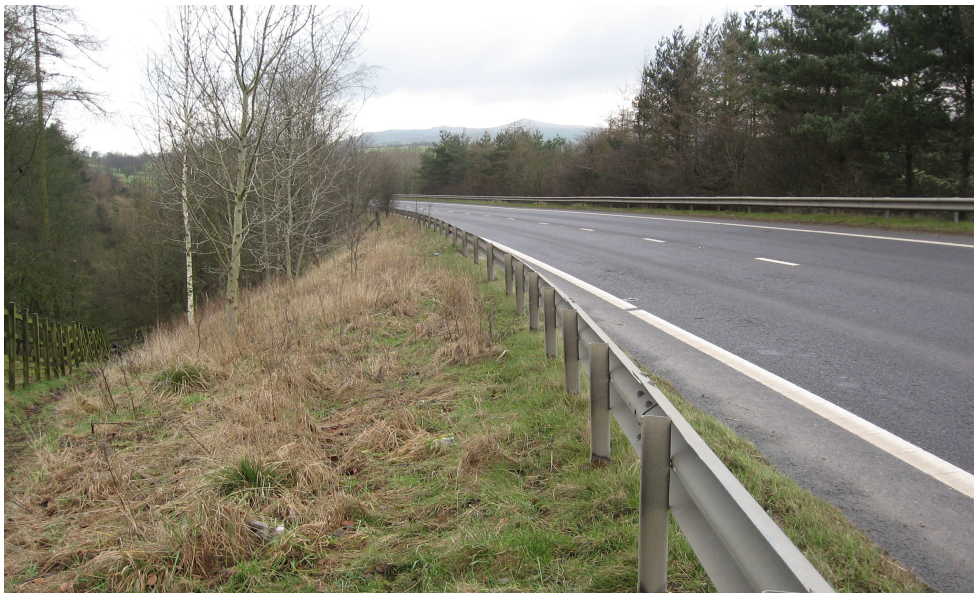
Figure 4 Crest of road embankment (Case History B) from left abutment
