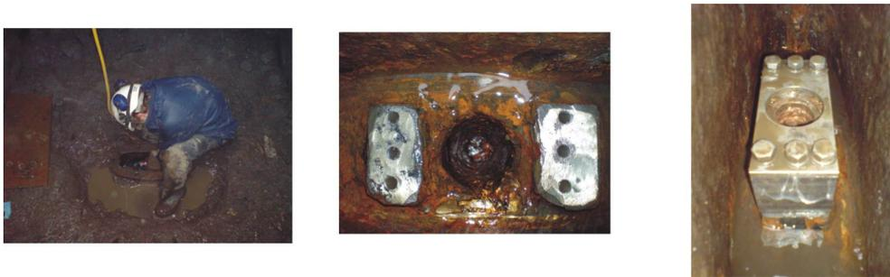
Figure 2: Valve gate prepared for attachment of new spindle nut carrier blocks
