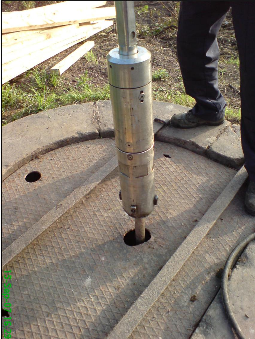
Figure 3: Typical H-Grip set up to release a seized valve
