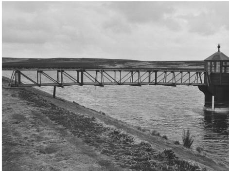
Fig. 6: Valve tower and Bridge
