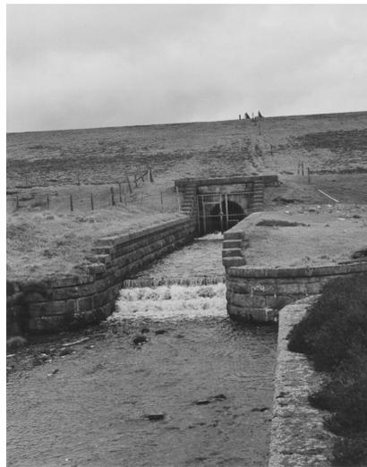
Fig 7: Masonry step overflow weir
