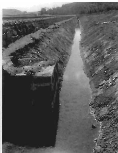
Fig. 13: Inlet diversion ditch
