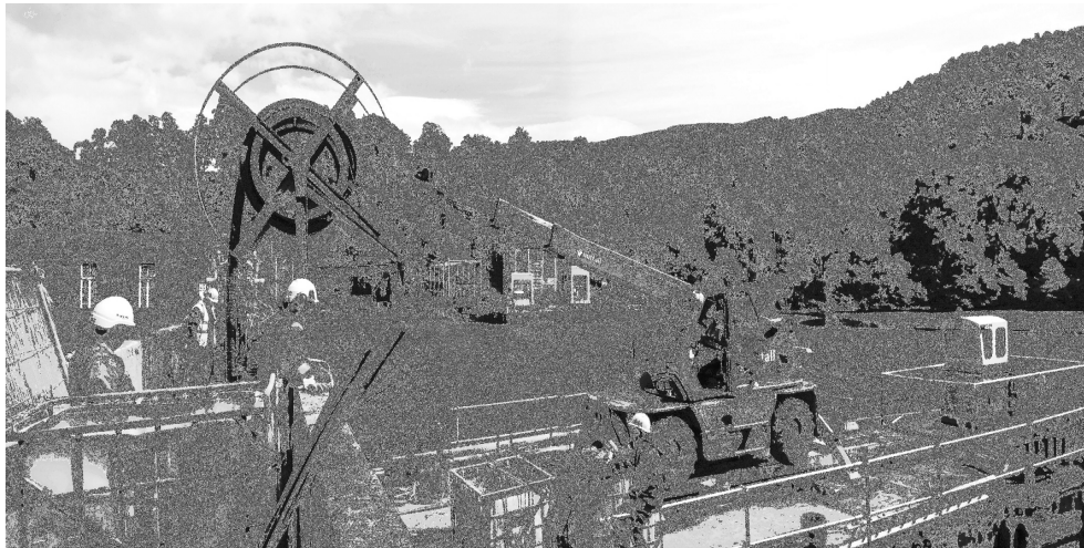
Figure 4 – Anchor installation using barge mounted telehandler
